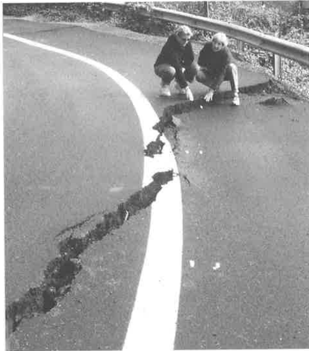
A 1982 evaluation by John Gentile, then at Oregon State University, pinpointed 153 prehistoric and present-day slides within a one-and-one-half-mile-wide strip between Roads End and Yachats in Lincoln County. The most susceptible unit was the clay-rich Nye Mudstone underlying marine terraces. Erosion of the Nestucca, Astoria, and Nye formations is particularly evident in this county, which is additionally subsiding relative to sea level. (Photo at Roads End; courtesy J. Orr)
