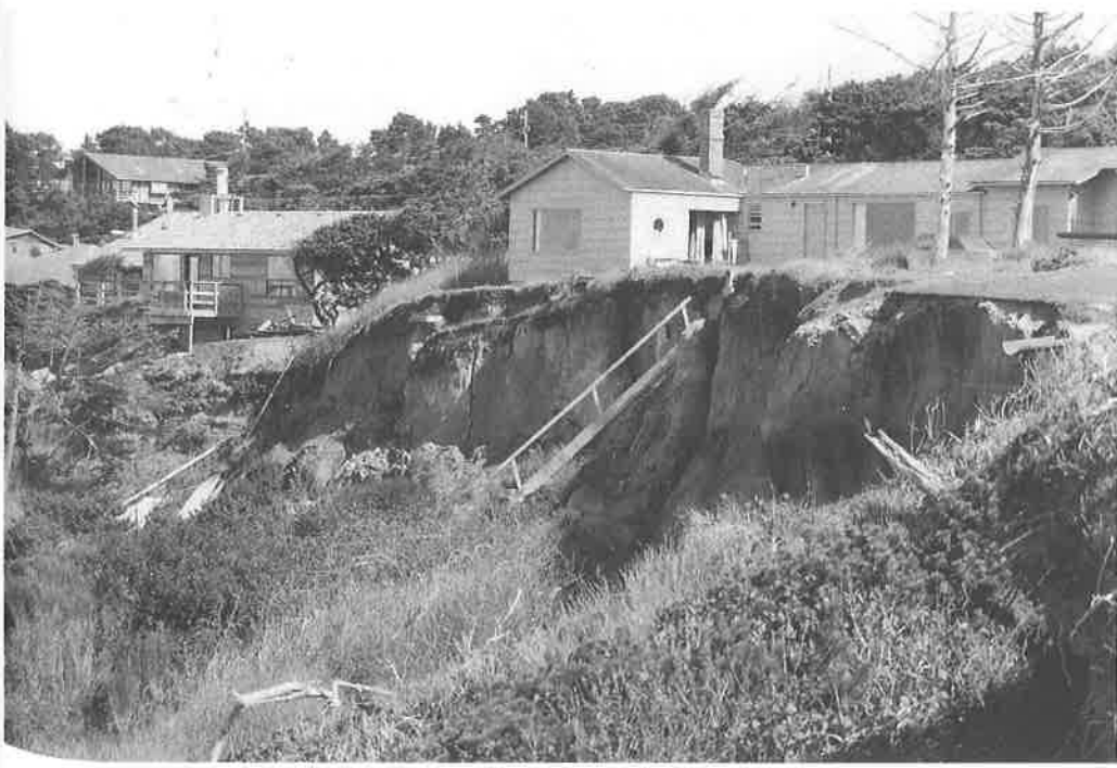
Newport has seen a remarkable combination of slumping, storm wave erosion, and landsliding that demolished the peninsula at Jump-Off Joe (above right) and moved the strand at Nye Beach inland as much as seven feet a year. The promontory and adjacent cliff are composed of poorly consolidated, seaward-dipping Astoria Formation and Nye Mudstones, topped by a terrace. Adjacent to Jump-Off Joe on 14th Street (left), an active slump block undercut housing in 1982. (The photos of Jump-Off Joe were taken in 1880, 1915, and 1926; courtesy Oregon Department of Geology and Mineral Industries)
