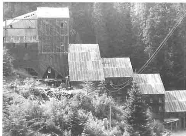
At the sophisticated Champion Mill, a 100 ton selective flotation plant processed ore in the Bohemia area. (Photo courtesy Oregon Department of Geology and Mineral Industries)
