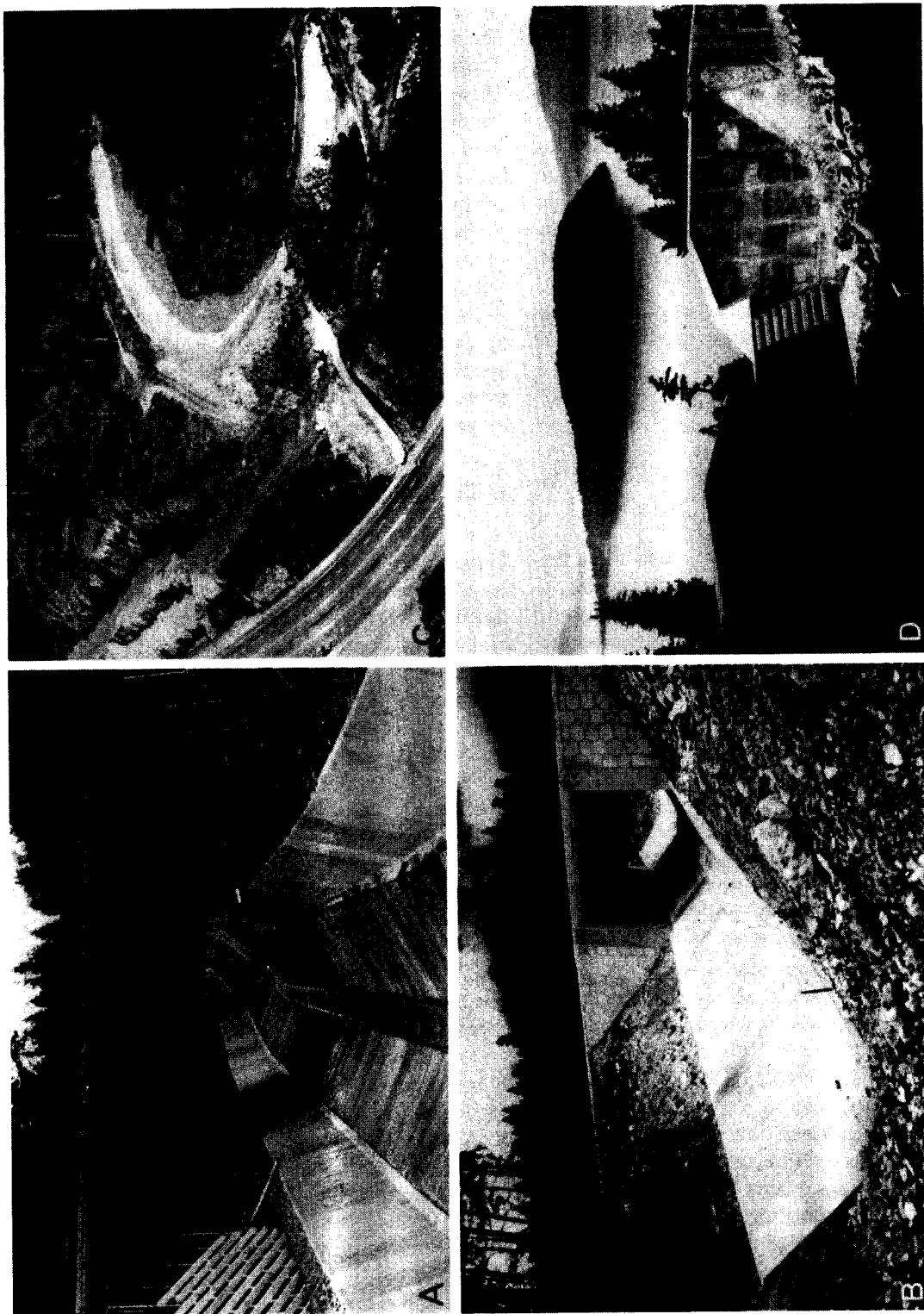
Figure 17.9. (A) Alberta Creek debris chute constructed after the February, 1983, debris-flow (Figure 17.4); (B) Bridge opening with debris chute; (C) Debris flow diversion dyke. A debris storage area of 12 500 m 3 capacity is created by a 5 m high dyke. The dark material within the dyke is the deposit of a debris-flow. Photograph courtesy of Thurber Consultants, Ltd. and Dr. Oldrich Hungr; (D) Debris interception barrier on Charles Creek. See Hungr et al. (1987) for a detailed description of the design. Photograph courtesy of Mr. Michael Younie
