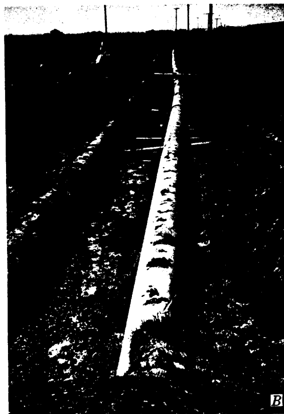
FIGURE 26.—Damage to a lined canal and oil pipelines caused by subsidence. A , Subsidence of part of a concrete-lined irrigation ditch; B , oil pipelines downwarped by subsidence.
