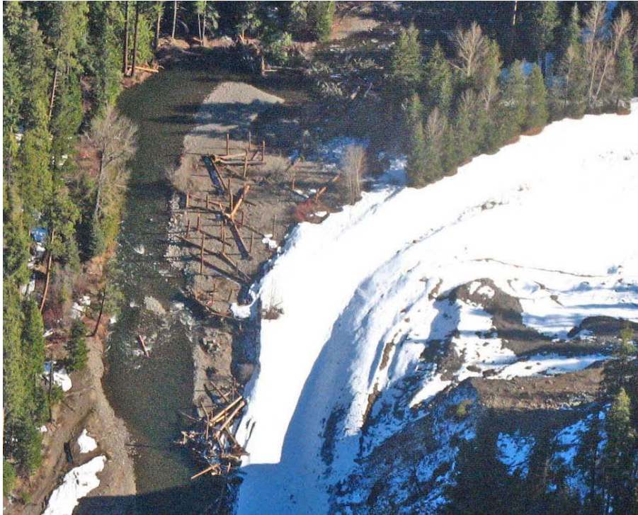
Figure 15. Floodplain wood placed on a constructed bar to roughen the former active channel where it previously abutted a rip-rap roadbed. The logs are braced against and attached to vertical log pilings (Klickitat River, WA, Inter-Fluve, Inc.).
