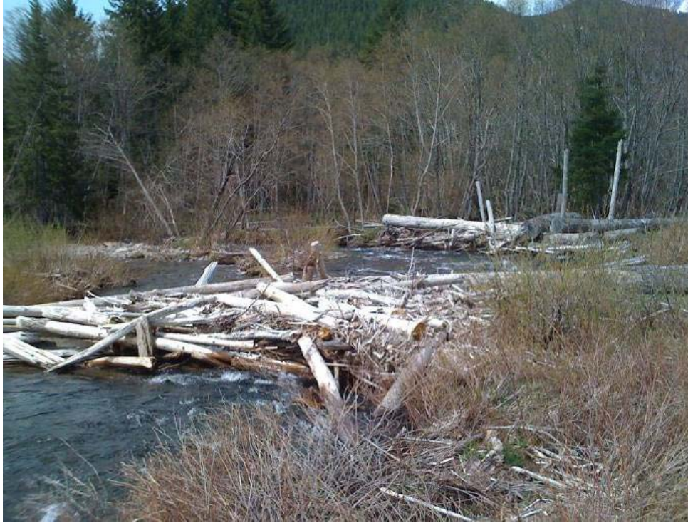
Figure 19. Log jam constructed in 2007. Photo taken 2 years after construction and after a 5-year return interval flood event (West Fork Hood River, OR, Inter-Fluve, Inc.).
