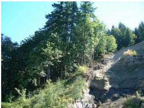
(c) Deep-seated landslide
