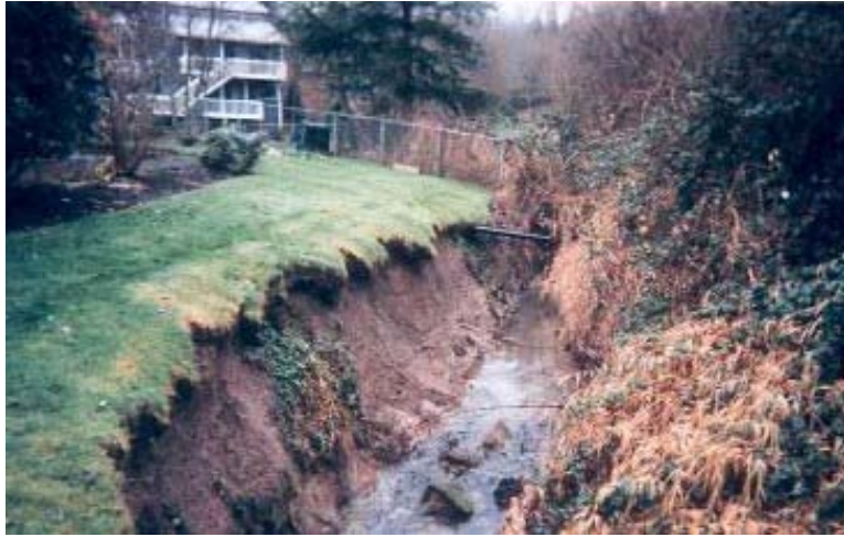
Figure 22. Channel incision. An example of channel instability in an incising channel. Columbia Creek, Oregon. Note undercut banks below rooting zone on left. Photo provided courtesy of Inter Fluve, Inc.
