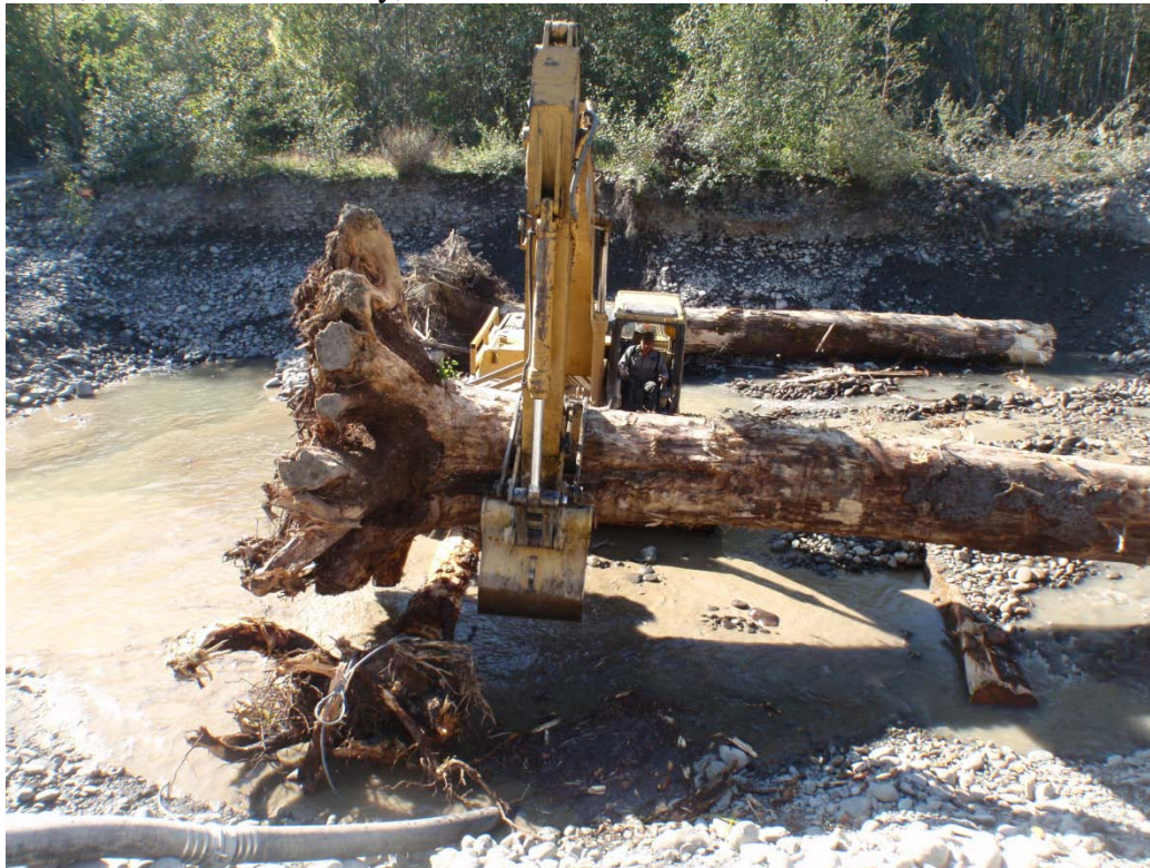
Figure 16. Use of large key pieces and additional stacked logs to increase stability (Elwha River, WA, Mike McHenry, Lower Elwha Klallam Tribe.).
