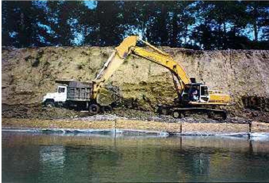
Figure 3. Construction platform for major streambank restoration, Little Miami River, Ohio. Source: Inter-Fluve, Inc.
