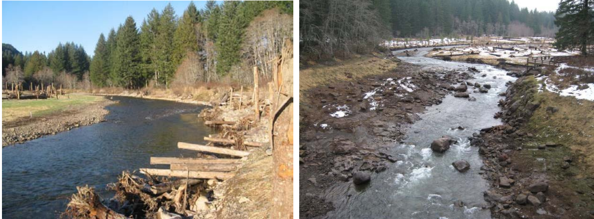
Figure 12. Reconstructed channel segments in the former reservoir of Hemlock Dam; Trout Creek, WA (Inter-Fluve, Inc.).
