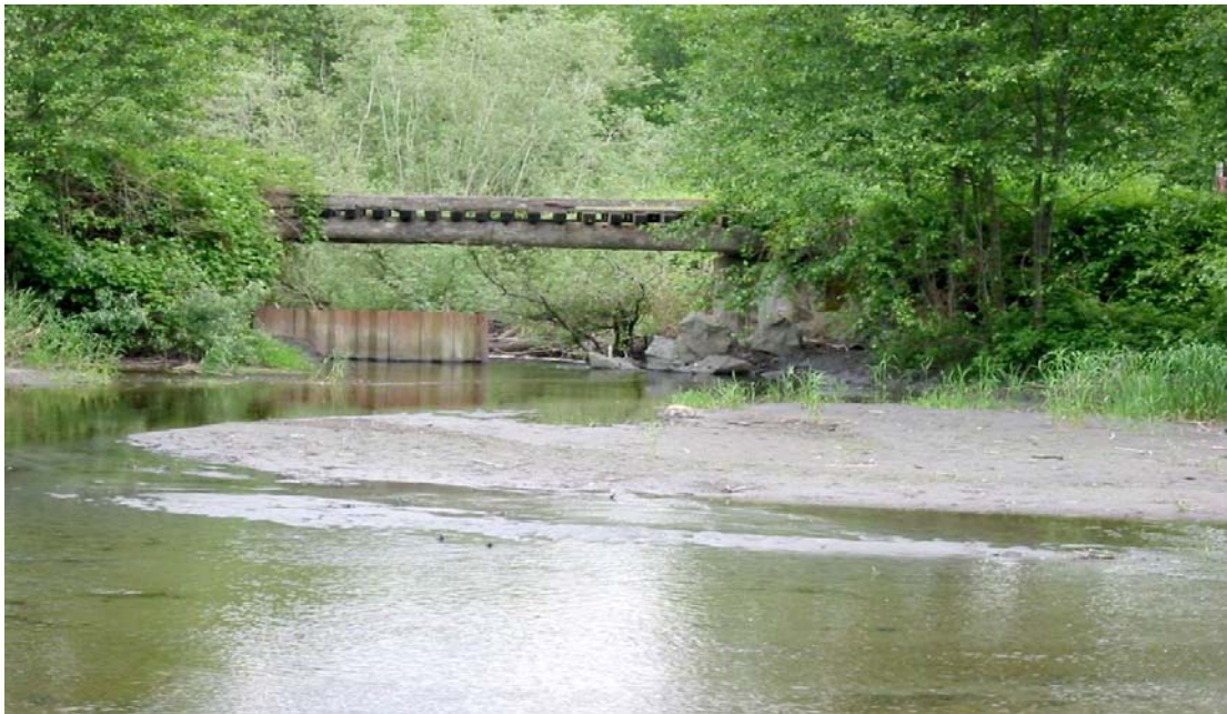
Instream Sediment Detention Basins Figure 4: Hansen Creek sediment basin, Skagit County. Looking downstream at outlet structure. Outlet is more ad hoc than other basins and can be a passage problem at some flows. Basin is actually many acres with only the outlet shown here.
