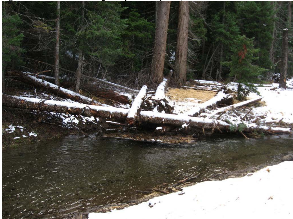
Figure 12. Constructed log complex in a pool (Klickitat River, WA, Inter-Fluve, Inc.).
