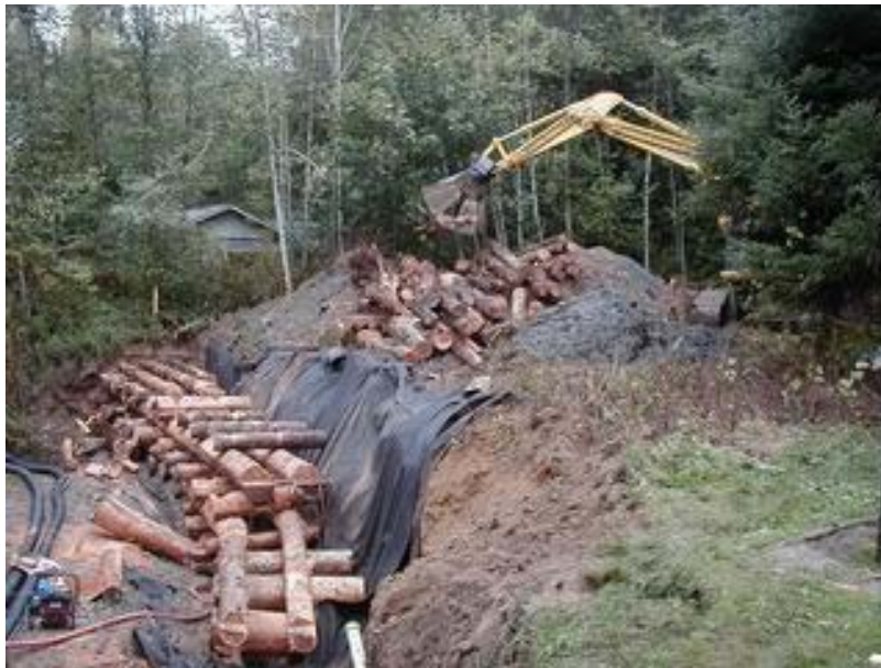
Figure 4. Stockpiling logs and soils on Beaver Creek. Source: Inter-Fluve, Inc.
