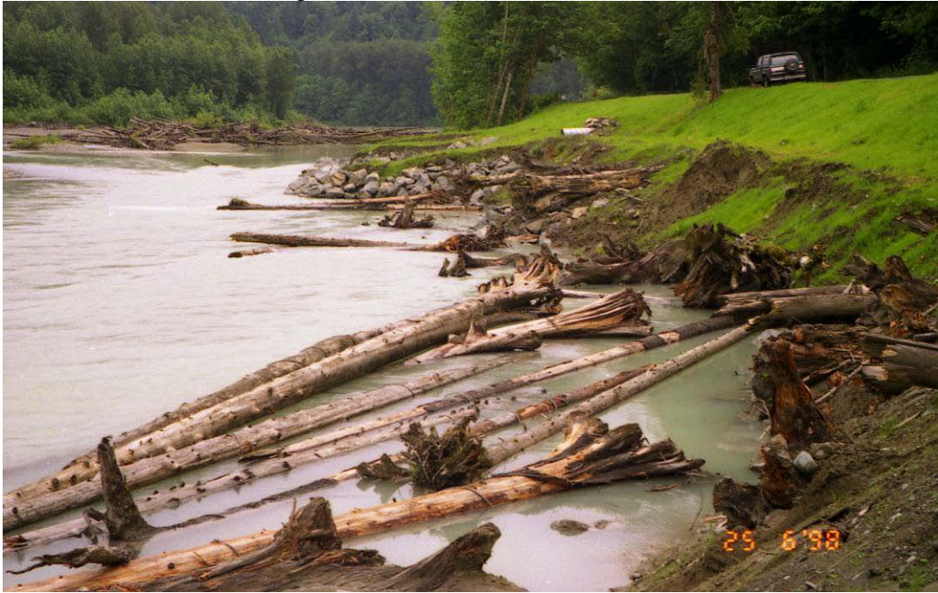
Figure 6. Large wood tethered on long cables to large drilled boulders (Sauk River side channel near SR 530, Skagit Co., WA).
