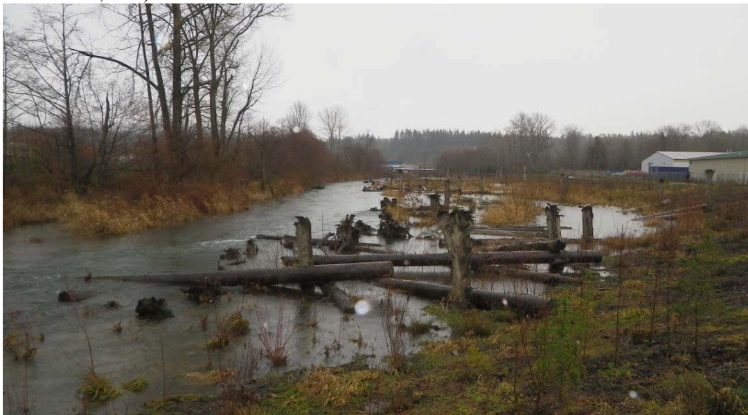
Figure 3. Large wood in stream, in overflow channel and on floodplain (Whatcom Creek, WA Inter-Fluve, Inc.)
