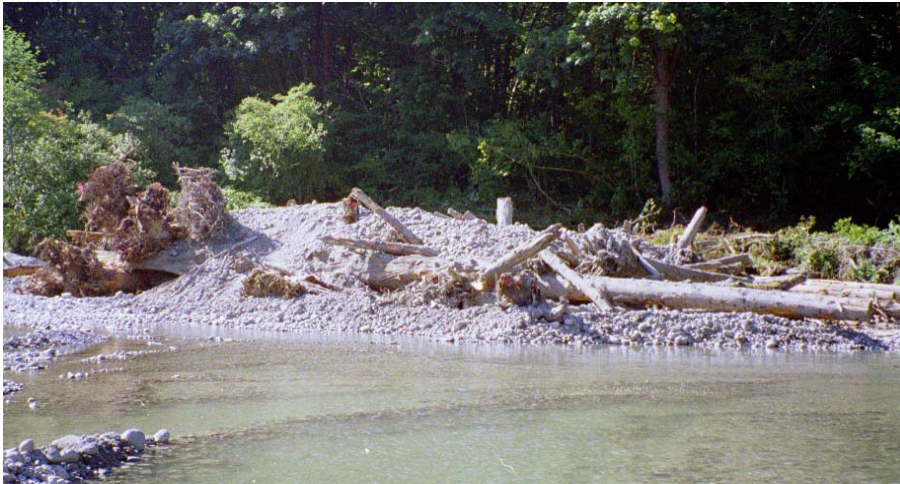
Figure 5. Log jam using gravel ballast (North Fork Stilliguamish River, Snohomish Co., WA).
