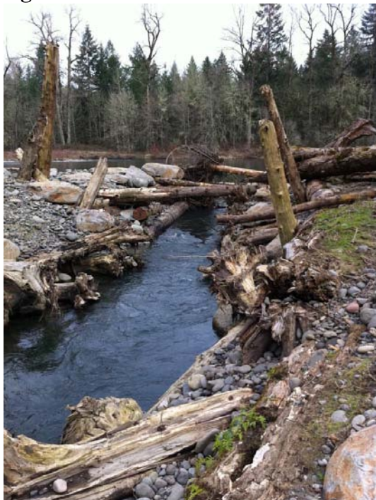
Figure 4. Constructed Side Channel Entrance (Clackamas River, OR, Inter-Fluve, Inc.).
