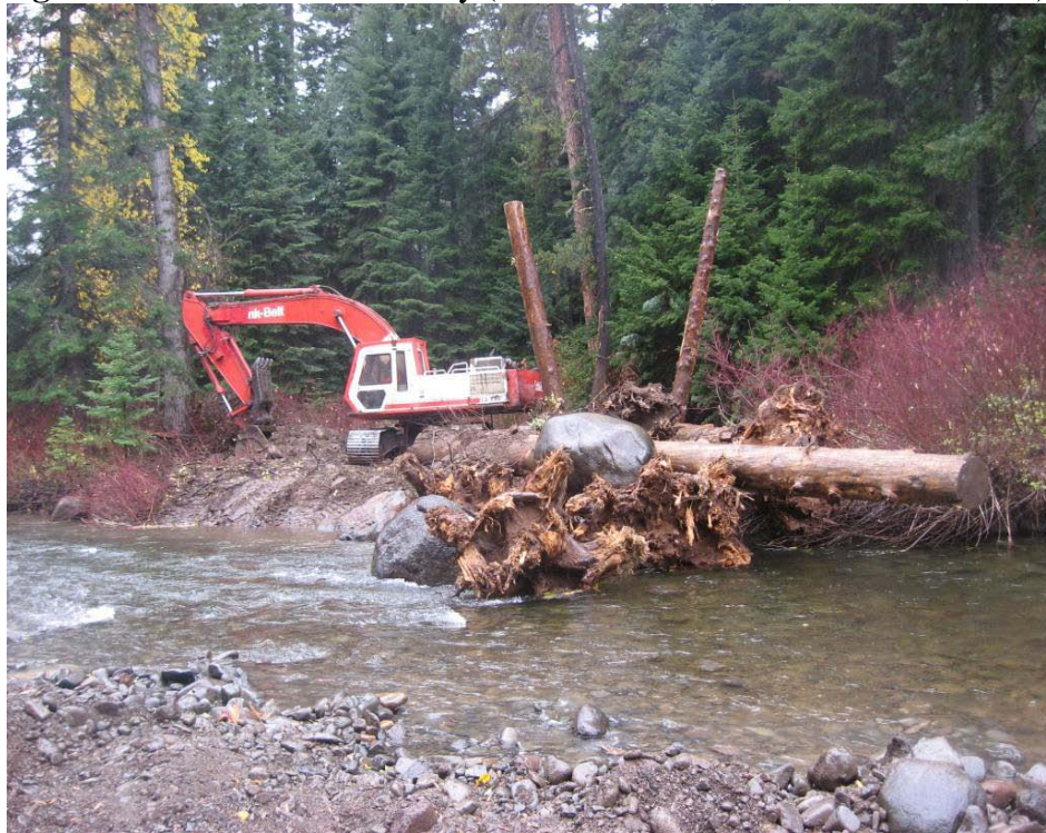
Figure 18. Boulders for stability (Klickitat River, WA, Inter-Fluve, Inc.).
