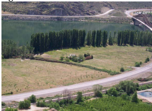
(a) Channel straightening
