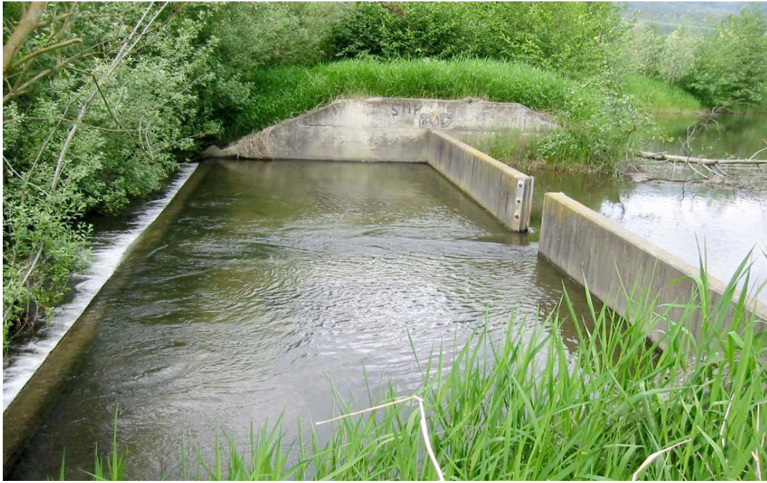
Instream Sediment Detention Basins Figure 3: Coal Creek sediment basin, detail of outlet structure. Downstream weir prevents erosion of channel. A more fish-friendly structure downstream of the slot might be a porous weir. Fish passage is an important consideration in the design of outlet structures.
