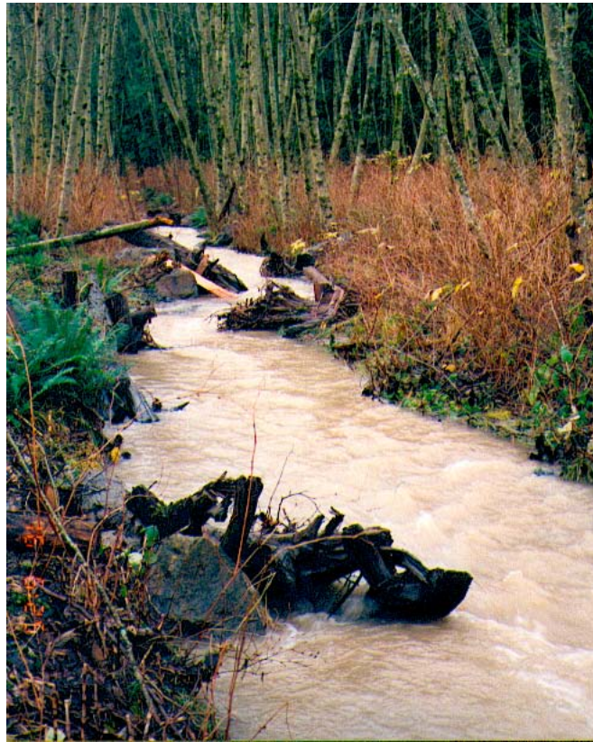
Figure 22. Constructed Log Complexes on Klahowya Creek, Skagit County, Washington. (Source: Robison, E. G. and R. Beschta. 1990. Characteristics of coarse woody debris in several coastal streams in southwest Alaska, USA. Canadian Journal of Fisheries and Aquatic Science 47:1684-93.)
