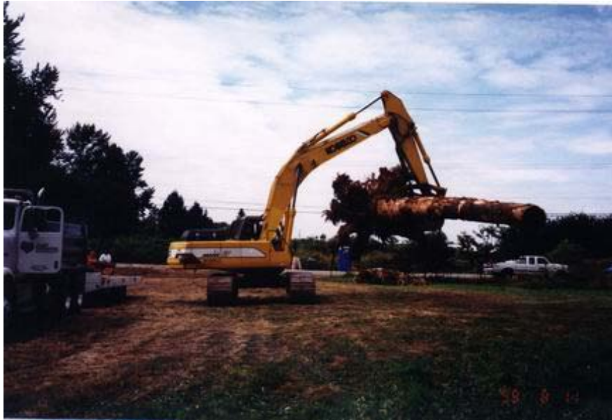
Figure 8. A track hoe excavator manipulating a large root wad and bole. Source: Inter-Fluve, Inc.
