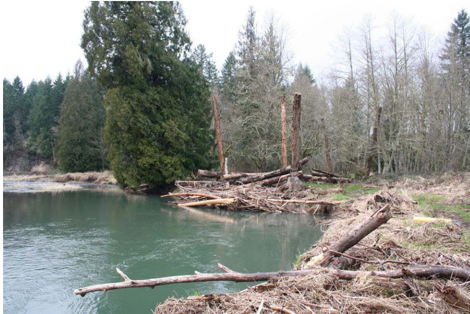
Figure 17. Collection of additional wood on a constructed meander bend log jam (Clear Creek, OR, Inter-Fluve, Inc.).
