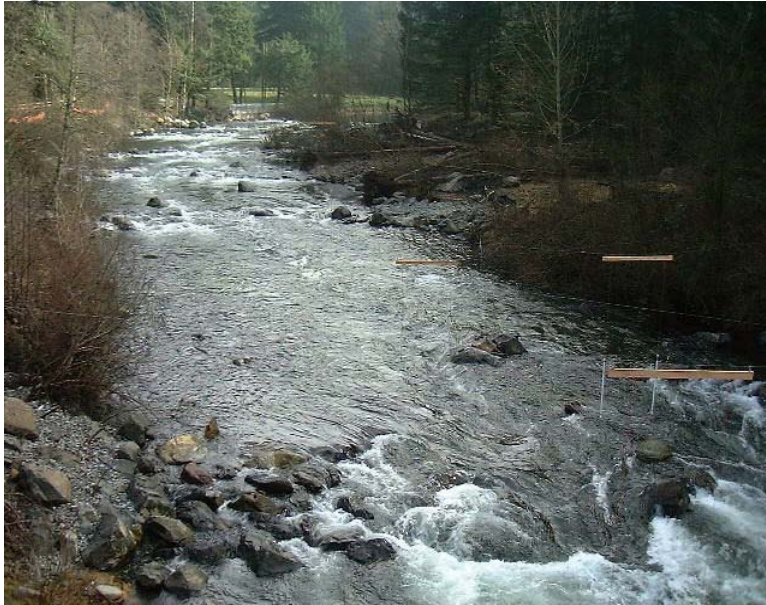
Figure 4. Porous boulder weir. Cedar River, WA.
