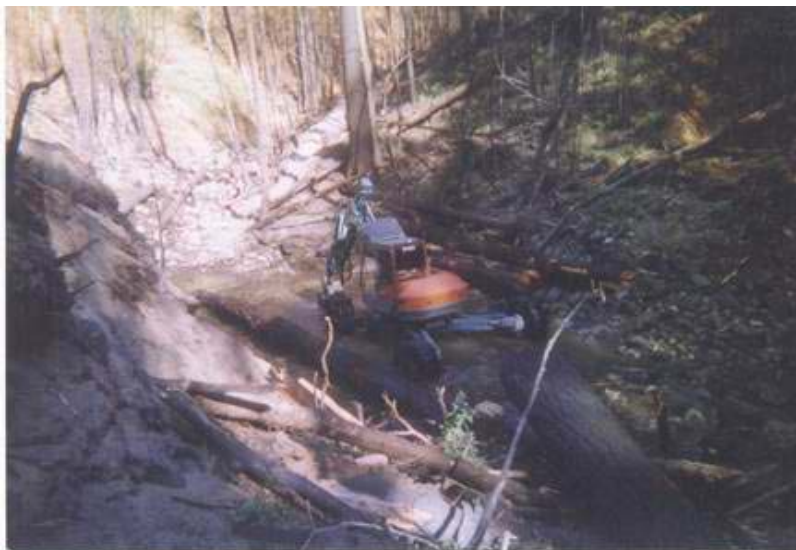
Figure 2. Spider Excavator placing rocks and logs in Whatcom Creek. Source: Inter-Fluve, Inc.
