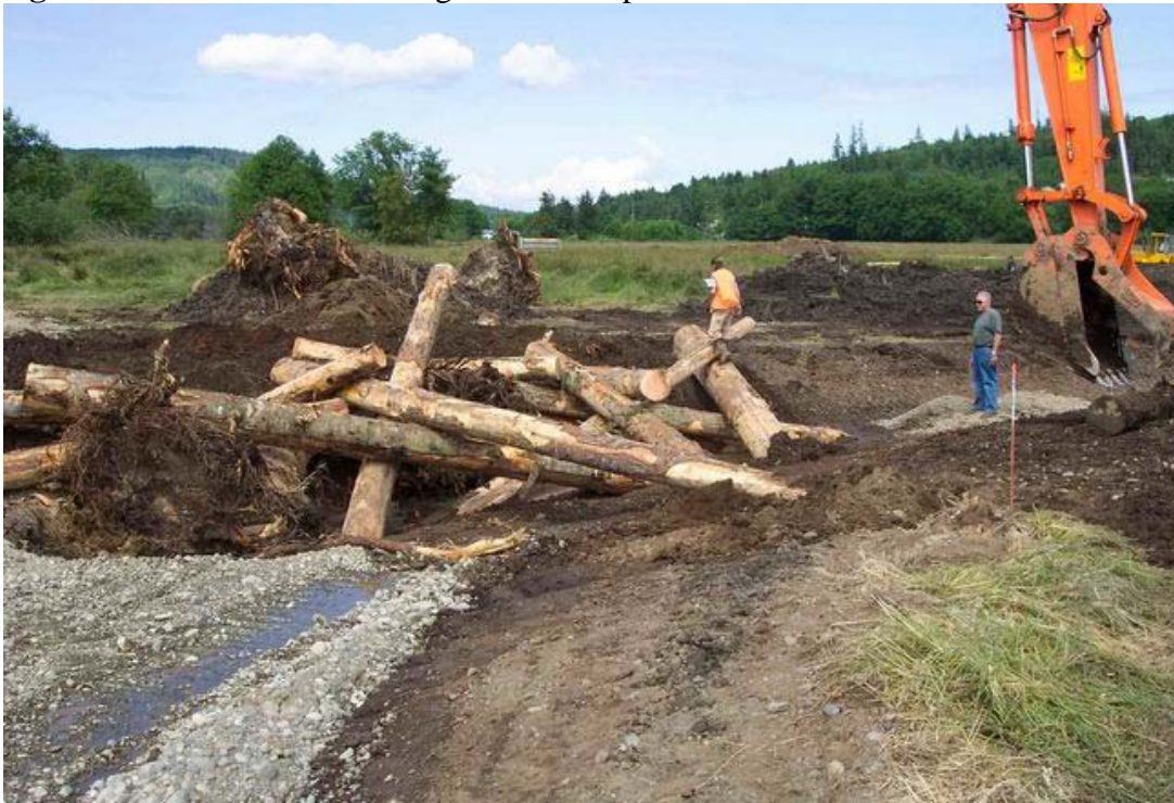
Figure 4. Construction of a large wood complex.
