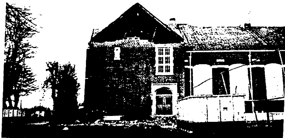
Fallen brick gable at Molalla High School resulting from the earthquake in northwestern Oregon on March 25, 1993.
