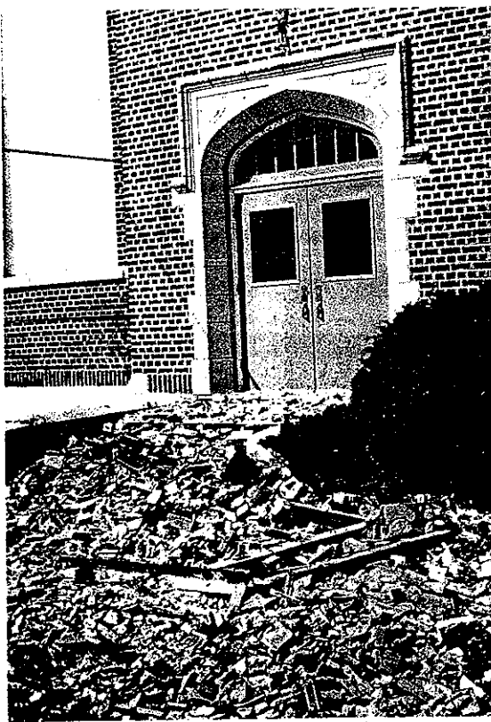
Figure 3 Damage to Molalla High School, Molalla, Oregon, from Scotts Mills earthquake of 1993. Left: Bricks from the unreinforced masonry gable over the doorway fell to the steps and sidewalk during the earthquake, illustrating the need for seismic strengthening of the structure. Top: The damage to the steps was revealed when the debris was removed.
