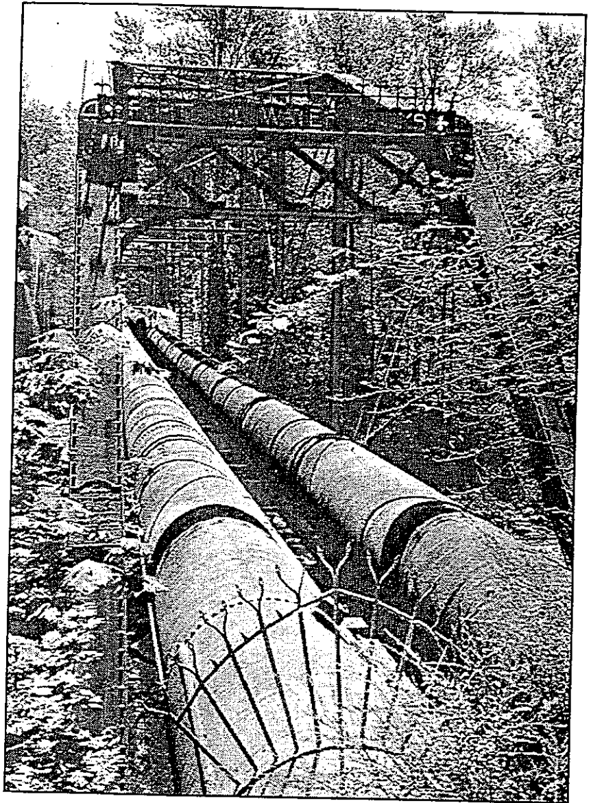
Portland's emergency water supply is delivered to the reservoir through these conduits on a bridge crossing the Sandy River. The bridge is also susceptible to damage from liquefaction and lateral spreading.
