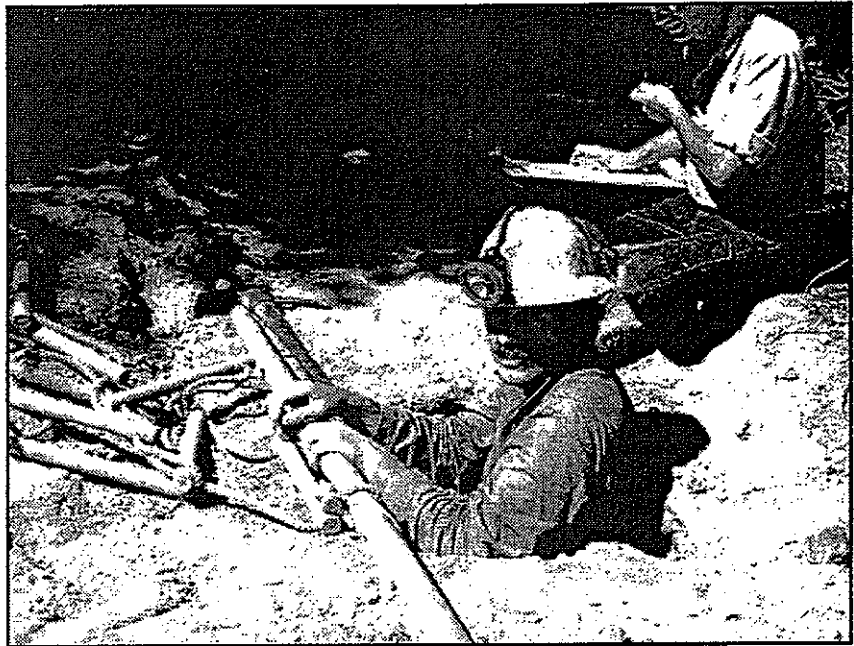
This geologist has just read a bore hole. Sometimes, subsurface investigation is needed to obtain sufficient information about site conditions to ensure safe development.
