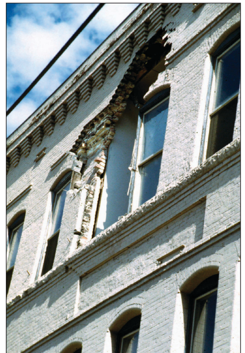
Figure 12. Partial collapse of URM building wall, Sodo neighborhood of Seattle.
