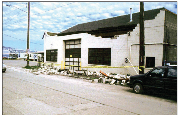
Figure 12. Partial collapse of URM building wall, Sodo neighborhood of Seattle.
