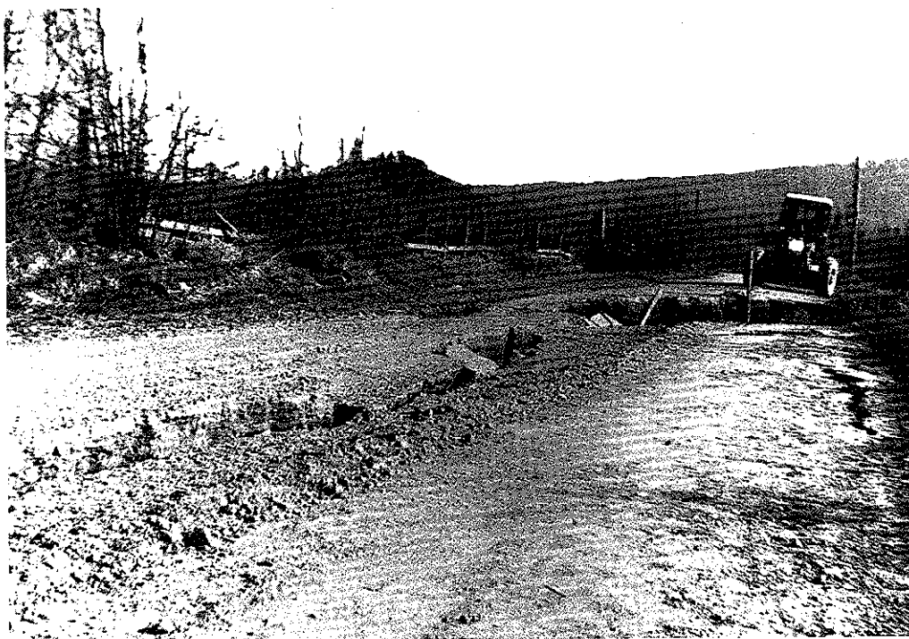
Figure 209. Slump in a 1- to 1.2-m-high road embankment in the Cowlitz River Valley, about 1.6 km southwest of Randle, Wash. (pl. 6, loc. 118). This April 13, 1949, earthquake-induced ground failure occurred in artificial fill underlain by loose liquefiable sand. The earthquake also produced sand boils in an adjacent field. Photograph by Alice Peters, Randle, Wash.
