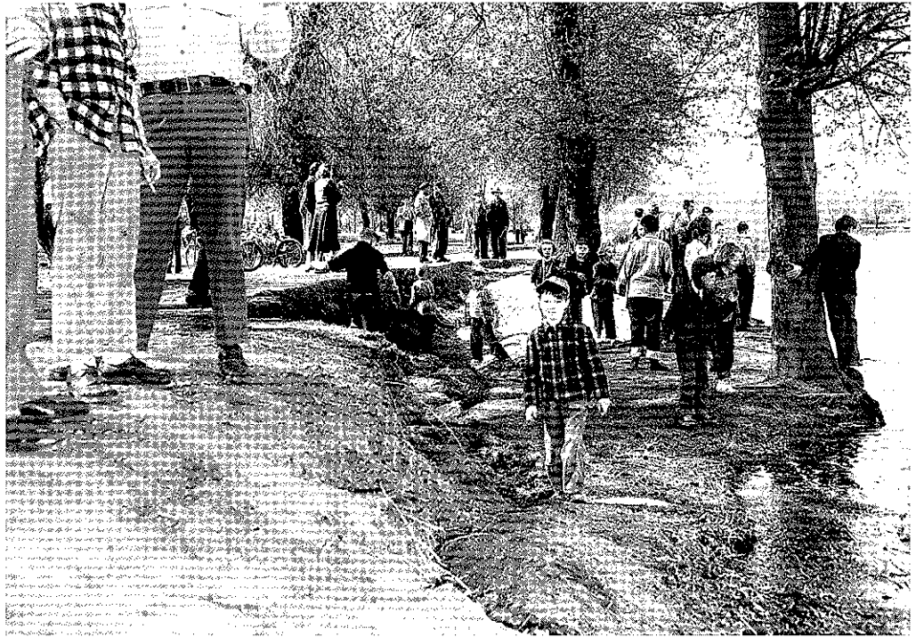
Figure 194. Slump along the shore of Green Lake, north of downtown Seattle. This 1949 earthquake-induced ground failure occurred near the south end of the lake (pl. 4, loc. 33) in an area that subsequently experienced ground failure during the April 29, 1965, earthquake. Photograph from the Seattle Post-Intelligencer Collection, courtesy of the Museum of History and Industry, Seattle, Wash.
