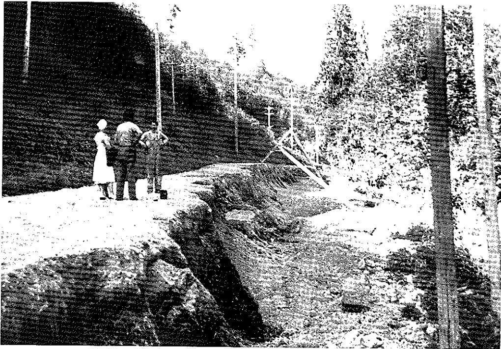
Figure 213. Scarp created by a landslide on the west side of Ohop Lake, Pierce County, Wash. (pl. 7, loc. 138). Incipient failure induced by the April 13, 1949, earthquake resulted in the development of a large ground crack. On May 13, complete failure occurred as the unstable mass suddenly slumped into the lake, damaging the roadway, utility lines, and cottages near the shore. Photograph used by permission of the Tacoma News Tribune.
