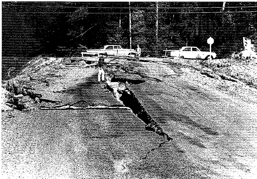
Figure 198. Damage to Country Club Road, southwest of Port Orchard, Wash. (pl. 4, loc. 2), due to slumping induced by the April 29, 1965, earthquake. This slump occurred in granular fill underlain by glacial deposits of the Vashon Drift. Photograph used by permission of the Bremerton Sun.
