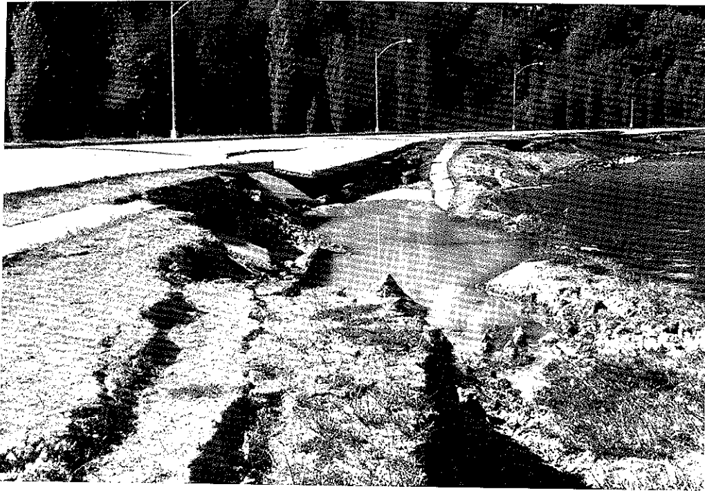
Figure 204. Damage to Deschutes Parkway, Olympia, Wash., resulting from a 1965 earthquake-induced ground failure (pl. 5, loc. 48). The parkway was constructed on granular fill placed on tidal flat muds that are now within the limits of Capitol Lake; failure was probably due to liquefaction. Photograph by Gerald W. Thorsen, Division of Geology and Earth Resources, Washington Department of Natural Resources, Olympia, Wash.
