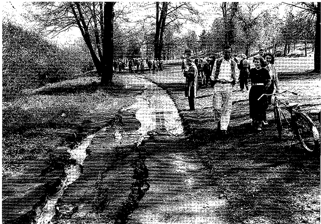
Figure 195. Ground cracks on the southeast side of Green Lake in north Seattle (pl. 4, loc. 33). The cracks opened during or shortly after the April 13, 1949, earthquake and probably resulted from subsidence and lateral movement of ground downslope toward the lake (out of sight to the left of view). Photograph from the Seattle Post-Intelligencer Collection, courtesy of the Museum of History and Industry, Seattle, Wash.
