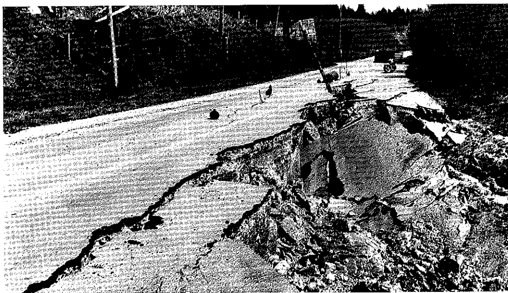
Figure 207. Damage to Black Lake Road south of Olympia, Wash. (pl. 5, loc. 44), caused by failure of a steep lake bank during the earthquake of April 13, 1949. Photograph used by permission of Jack Goldsby, Tumwater, Wash.
