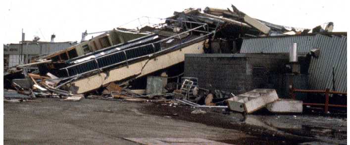
In 1964, the control tower at Anchorage, Alaska International Airport fell during the M9.2 earthquake. It was a split-level structure that was seven stories high on one side and built of reinforced concrete. Photo: USGS
