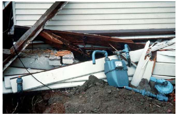
Houses don't need to collapse to be evacuated. This house shifted off its foundation in the 1989 Loma Prieta, California quake and now all the utilities are disconnected. Photo: H. G. Wilshire, USGS
