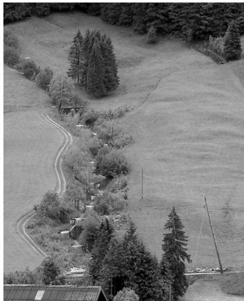
Fig. 7. (A) Upstream view of some of the numerous grade-control structures along the Vogelbach, a Swiss mountain stream, June 2004. (B) Upstream view of numerous grade-control structures along the Lumpenenbach, a Swiss mountain stream, June 2004.
