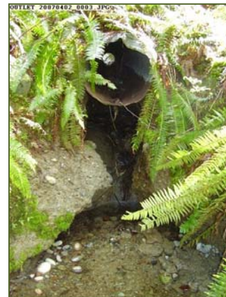
Photo 13: Fish Passage Barrier
