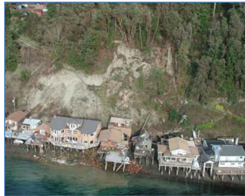
Photo 17: Salmon Beach Landslide, Tacoma
