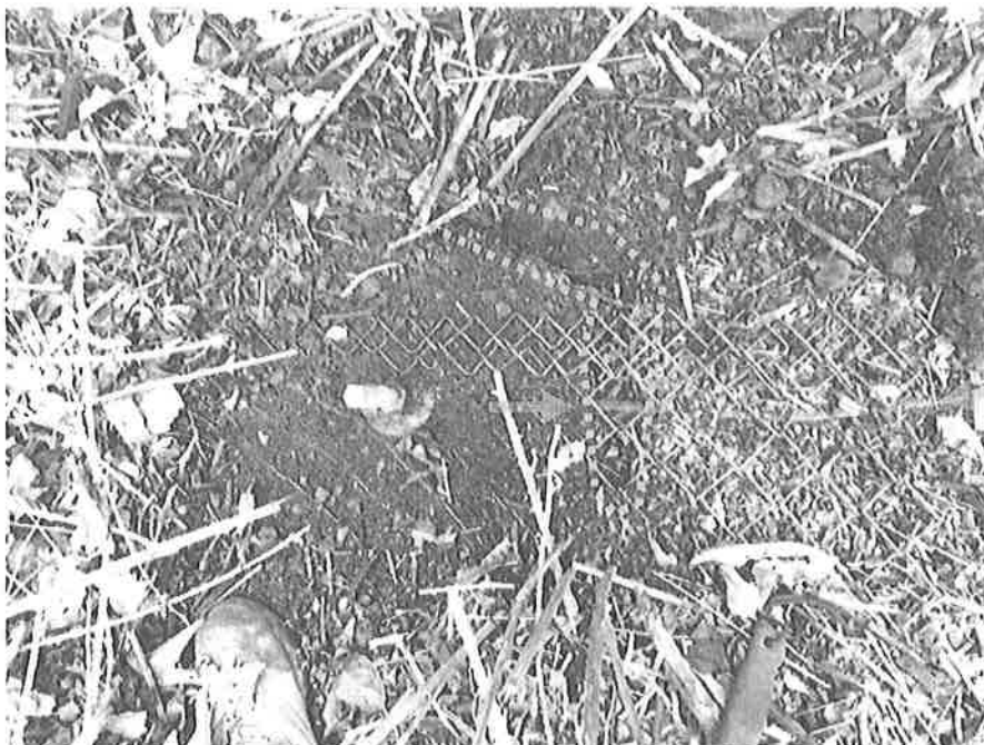
Rock anchor and top of draped mesh in area south of the 2014 rockslide.
