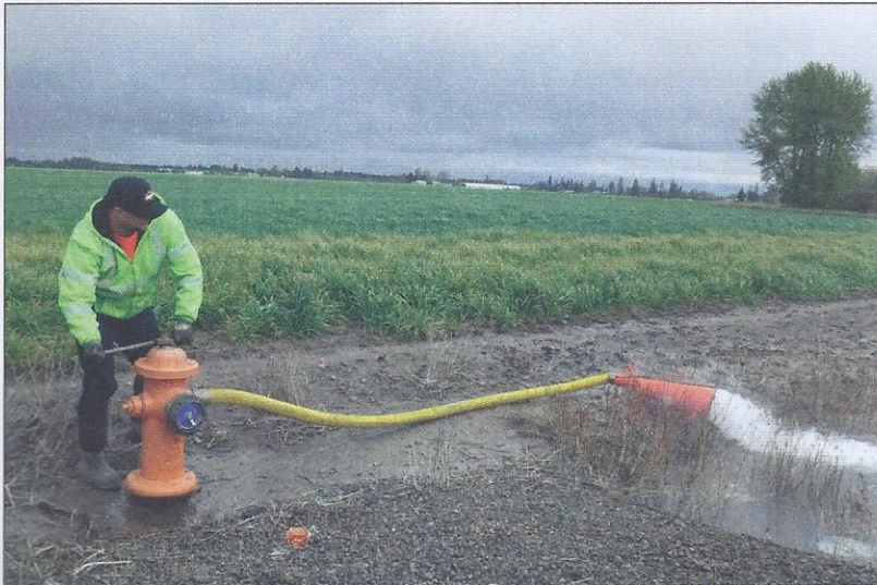
Distribution system operator Kyle Krake flushes water lines to maintain water quality
