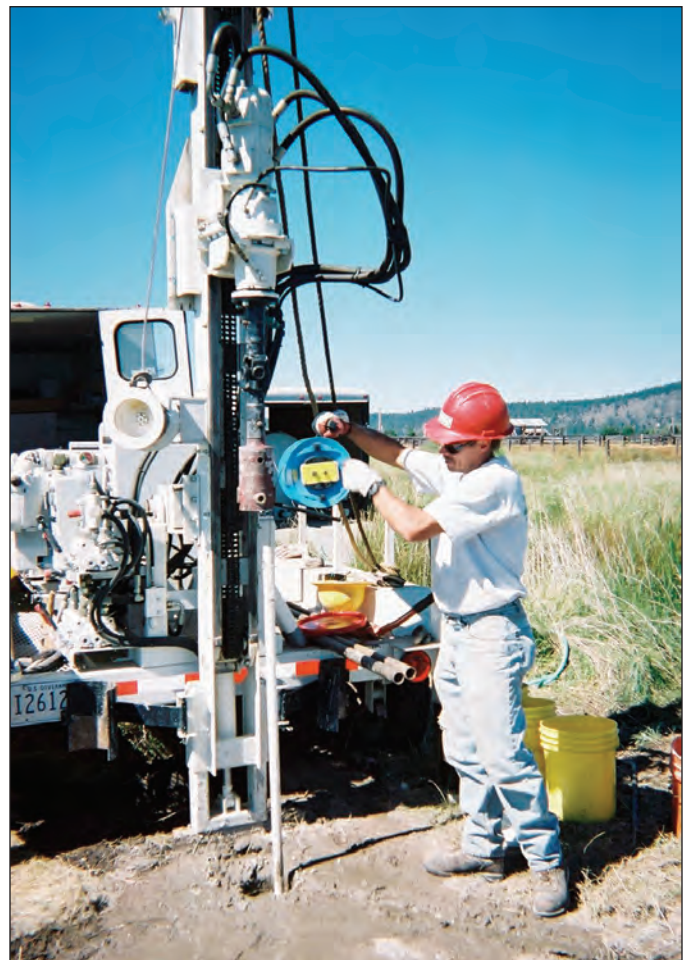
Construction of ground-water piezometers in the North Unit of the Wood River Wetland (looking north). Photograph taken by Charley Palmer, U.S. Geological Survey, August 2003.
