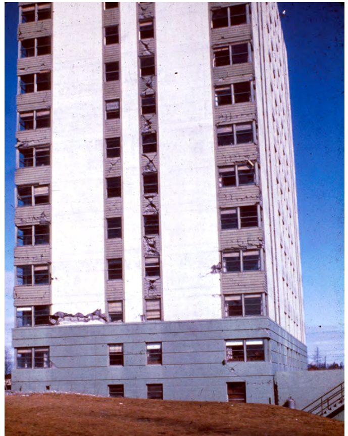
In the 1964 Alaska earthquake, this fourteen-story reinforced concrete apartment building in Anchorage was severely damaged by the ground shaking it endured. Photo: USGS
