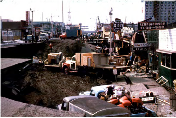
Before the earthquake, the sidewalk in front of these Anchorage stores on the right was at the level of the street on the left. Note that buildings and pavement not involved in the 11 foot (3 meter) landslide show little damage. Photo: USGS
