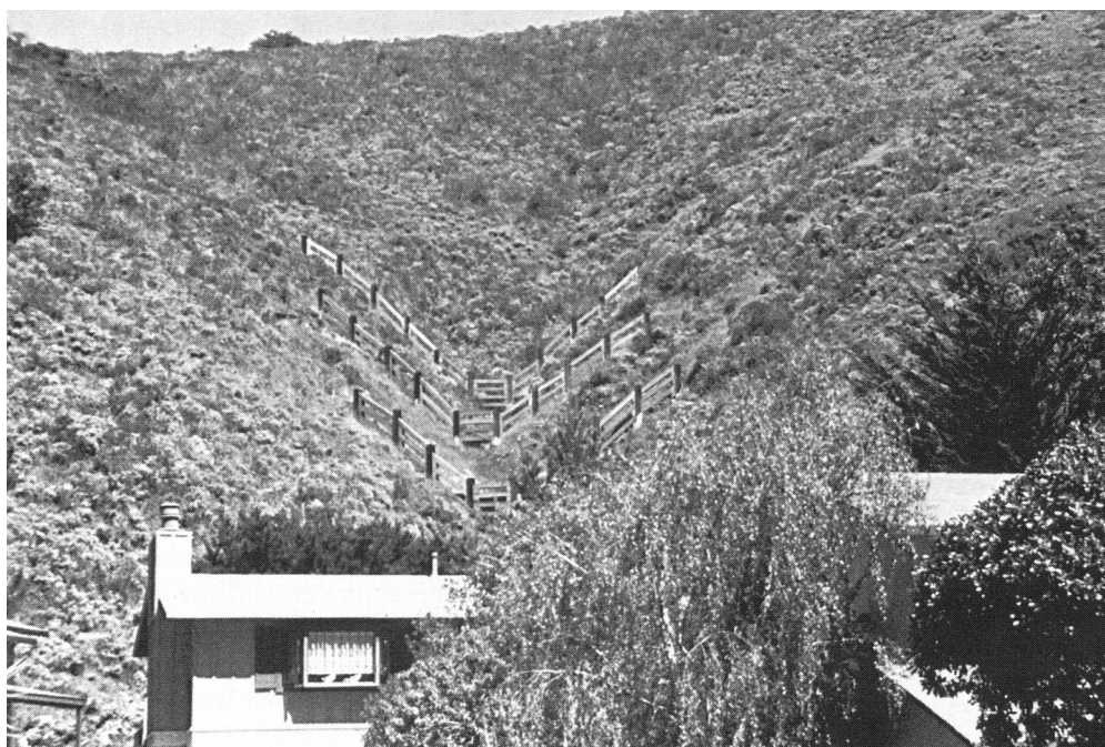
Figure 28. Debris fences installed below potential initiation sites in Pacifica, California. (From Montgomery and others, 1991)
