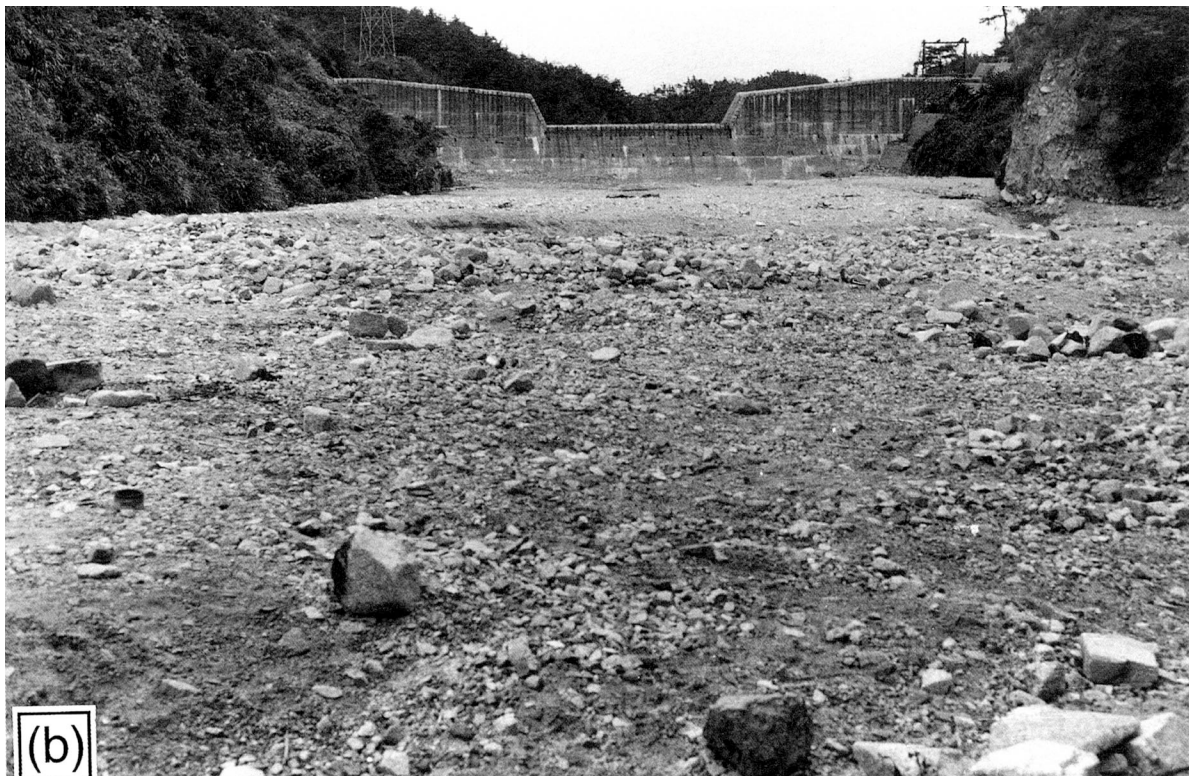
Figure 33. Check dam in Hyogo, Japan (30 m high, 78 m long, storage capacity 300,000 m 3 ), (a) before and (b) after a debris flow. (Photo from United Nations, 1996)
