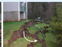
translational slide (most slides are combinations of translational and rotational movement)
