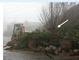
earth flow (unchanneled flow)
