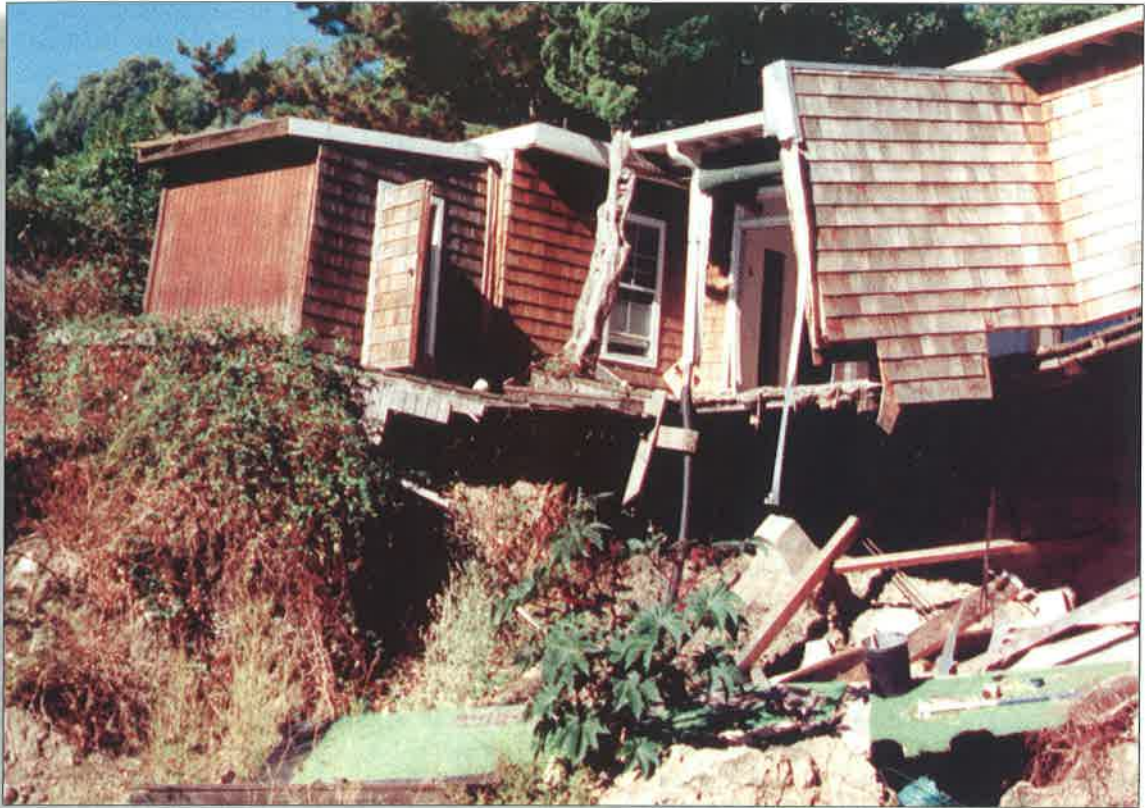
Reactivated prehistoric landslide destroyed this home in Southern California. (Edward A. Keller)
