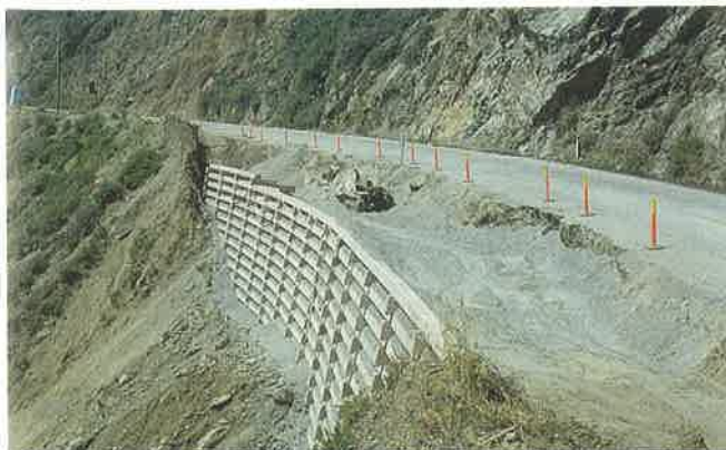
▲ FIGURE 6.19 Retaining wall (concrete cribbing) used to help stabilize a roadcut. (Edward A. Keller)
