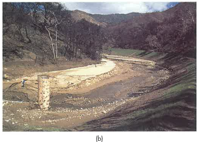
◀ FIGURE 5.19 (a) Comparison of runoff from a paved area through a storm drain with runoff from a paved area through a temporary storage site (retention pond). Notice that the paved area drained by way of the retention pond produces a lesser peak discharge and therefore is less likely to contribute to flooding of the stream. (Modified after U.S. Geological Survey Professional Paper 950.) (b) Photograph of a retention pond near Santa Barbara, California. (Edward A. Keller)
