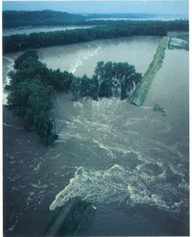
▲ FIGURE 5.30 Failure of this levee in Illinois during the 1993 floods of the Mississippi River caused flooding in the town of Valmeyer. (Comstock, Inc.)
