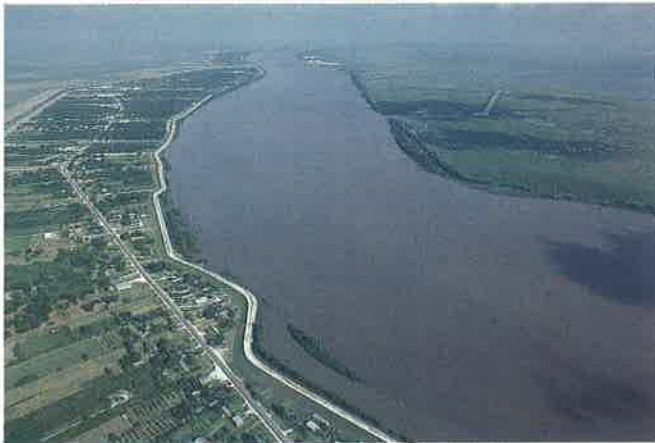
▲ FIGURE 5.18 Levee with a road on top of it protects the bank (left side of photograph) of the lower Mississippi River at this location in Louisiana. (Comstock, Inc.)
