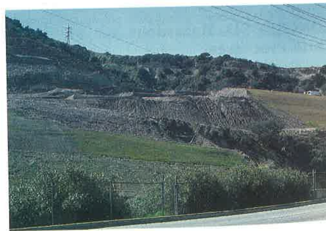
▲ FIGURE 1.11 Photo of soil erosion from human-constructed slope (Edward A. Keller)
