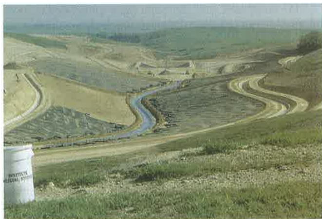
▲ FIGURE 12.5 Rock Creek municipal landfill, Calaveras County, California, under construction. The light brown slope in the central part of the photograph is a compacted clay liner. The sinuous ditch is part of the leachate collection system, and the square pond in the upper part of the photograph is the leachate evaporation pond under construction. (Courtesy of John Kramer)
