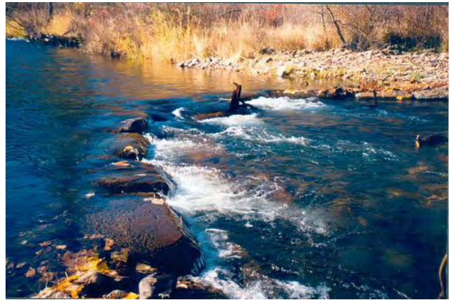
Porous Weirs Figure 5: Porous Cross Vane on stream in southeastern Washington.
