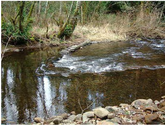
Porous Weirs Figure 4: Porous Cross Vane on Cedar Creek, Clark County, Washington.
