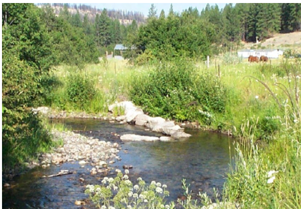
Porous Weirs Figure 6: J-Hook Rock Vane on Omak Creek, Okanogan County. Photo provided courtesy of the Natural Resources Conservation Service.
