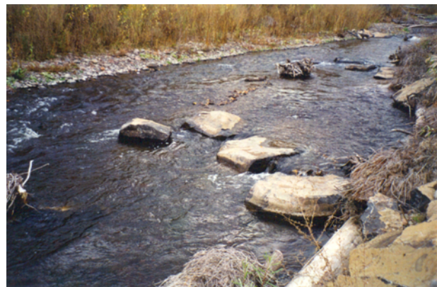
Porous Weirs Figure 7: J-Hook Rock Vane on stream in southeastern Washington.
