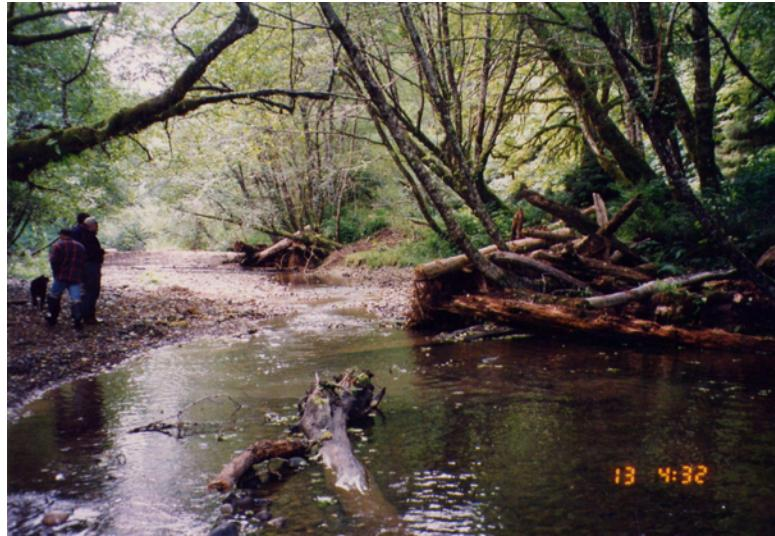
**Large Wood and Log Jams Figure 7.** LW complex on the Little Hoko River anchored by wedging LW between trees on the bank.
