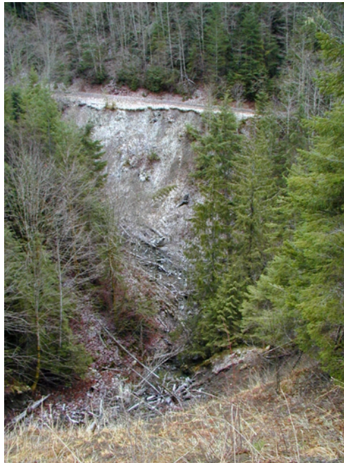
Figure 2.3. Erosion initiated by poor road drainage. Source: Paul Bakke
