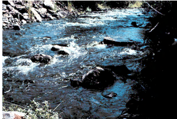
Boulder Clusters Figure 9: Constructed boulder clusters in the Tucannon River, Columbia County, Washington.
