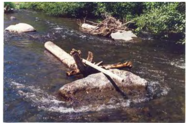
Boulder Clusters Figure 6: Constructed boulder cluster in Touchet River, Columbia County, Washington
