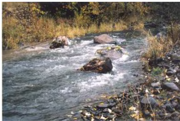
Boulder Clusters Figure 6: Constructed boulder cluster in Touchet River, Columbia County, Washington
