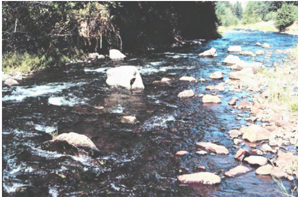
Boulder Clusters Figure 9: Constructed boulder clusters in the Tucannon River, Columbia County, Washington.
