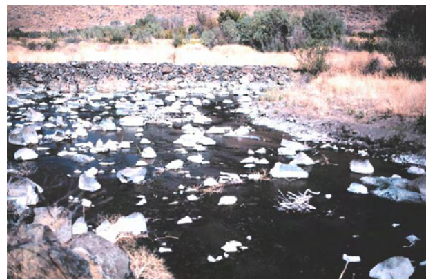
Boulder Clusters Figure 11: Constructed boulder clusters in Murderers Creek.
