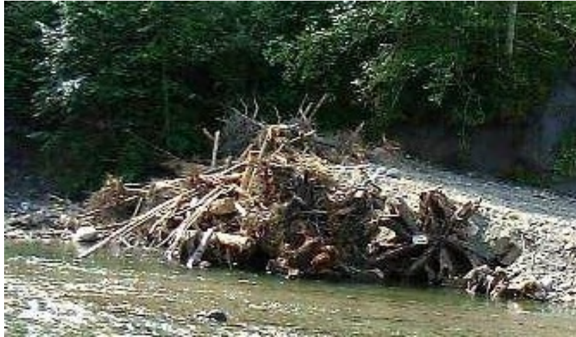
Figure 1 North Fork Stilliguamish River, Snohomish Co., log jam using gravel ballast.
