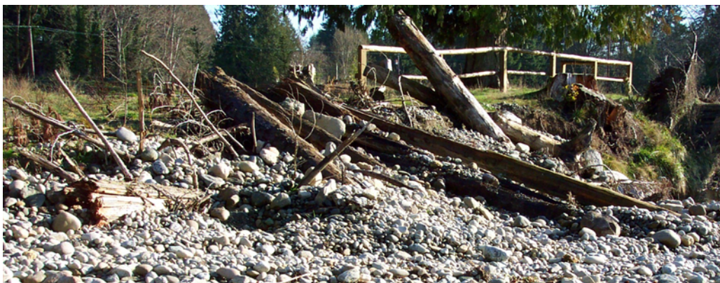
Figure 3 Gorst Ck., Kitsap Co., log bank protection using gravel ballast.
