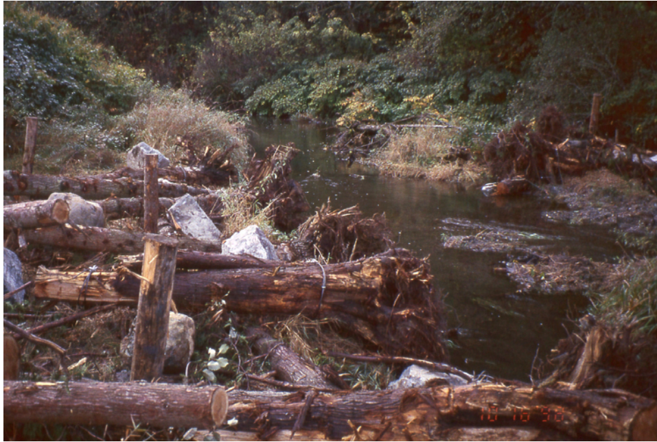
Figure 8 Samish River, Skagit Co. Large wood anchored using a combination of techniques; rock ballast, cabling, and pilings.
