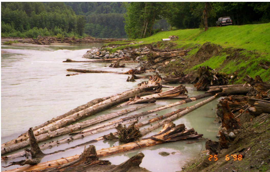
Figure 7 Sauk River side channel near SR 530, Skagit co. Large wood tethered on long cables to large drilled boulders.
