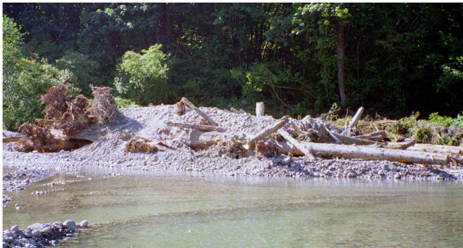
Figure 2 North Fork Stilliguamish River, Snohomish Co., log jam using gravel ballast.
