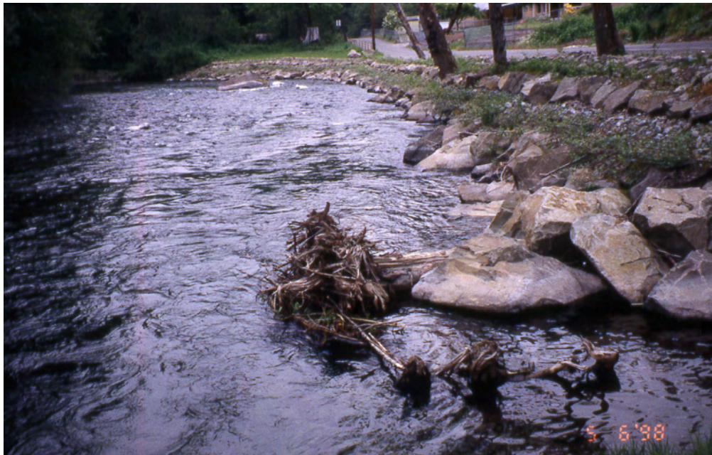
Figure 9 Cedar River, Darre Dam project, King Co. Large wood anchored in groin.
