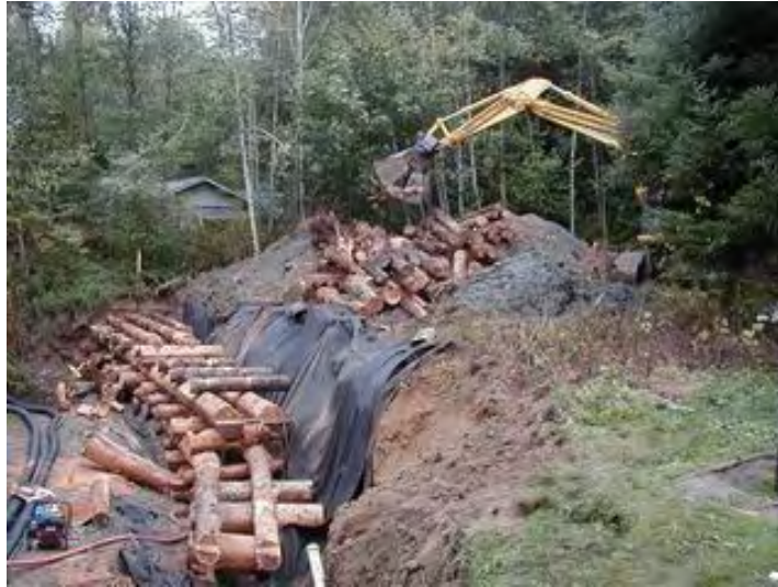
Construction Considerations Figure 4. Stockpiling logs and soils on Beaver Creek. Source: Inter-Fluve, Inc.
