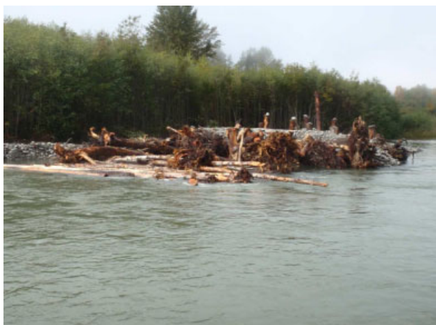
Figure 2. Photograph of a typical engineered log jam on the Elwha River, Washington State, USA. This figure is available in colour online at wileyonlinelibrary.com
