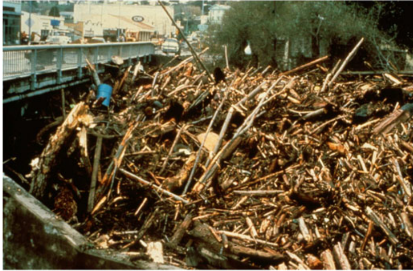
Figure 2. Logjam upstream of the Soquel Drive Bridge (Soquel, California, USA) after January 1982 storm. For scale, note oil drum (1 m height by 0.66 m width) entangled in logjam in upper left of photograph (photo taken by Gerald Webber, used with permission). This figure is available in colour online at wileyonlinelibrary.com/journal/rra .
