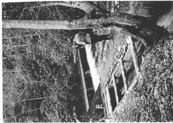
Figure 1.2 Forge Creek Dam in Cades Cove, in eastern Tennessee, is an example of a small, run-of-river structure. This view looks upstream from the west bank of the head-race and shows the main and diversion dams. A small diversion canal that supplied water to a mill is on the left. Courtesy of the Library of Congress, Prints and Photographs Division, Historic American Buildings Survey, Reproduction Number 5-CADCO, 1-24.
