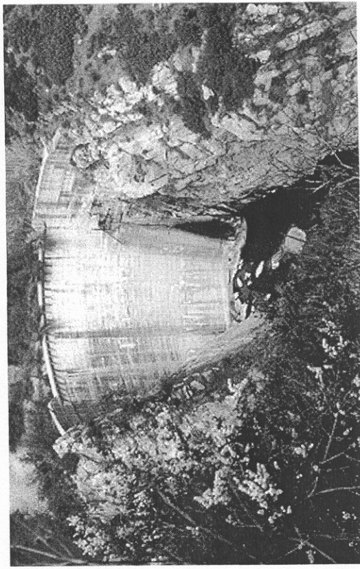
Figure 1.6 Rindge Dam, built in the 1920s on Malibu Creek in California, is an example of a concrete arch dam. Courtesy of Sarah Baish.
