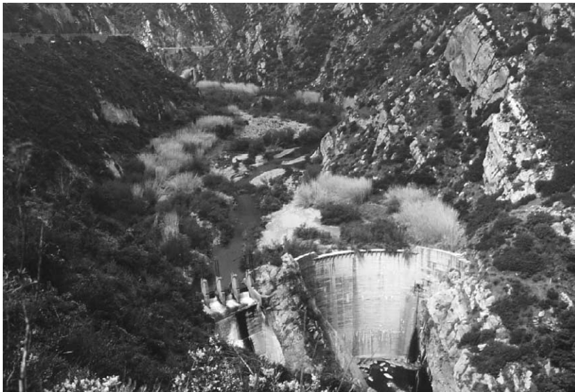
Fig. 11. Rindge Dam, Malibu Creek, Calif., is a candidate for removal. The dam is 60 m (100 ft) high and has a reservoir filled with sediment. Photo by Sarah Baish, Heinz Center.
