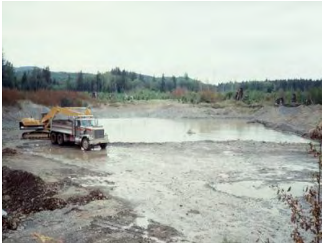
(b) Dismal Pond site during construction.
