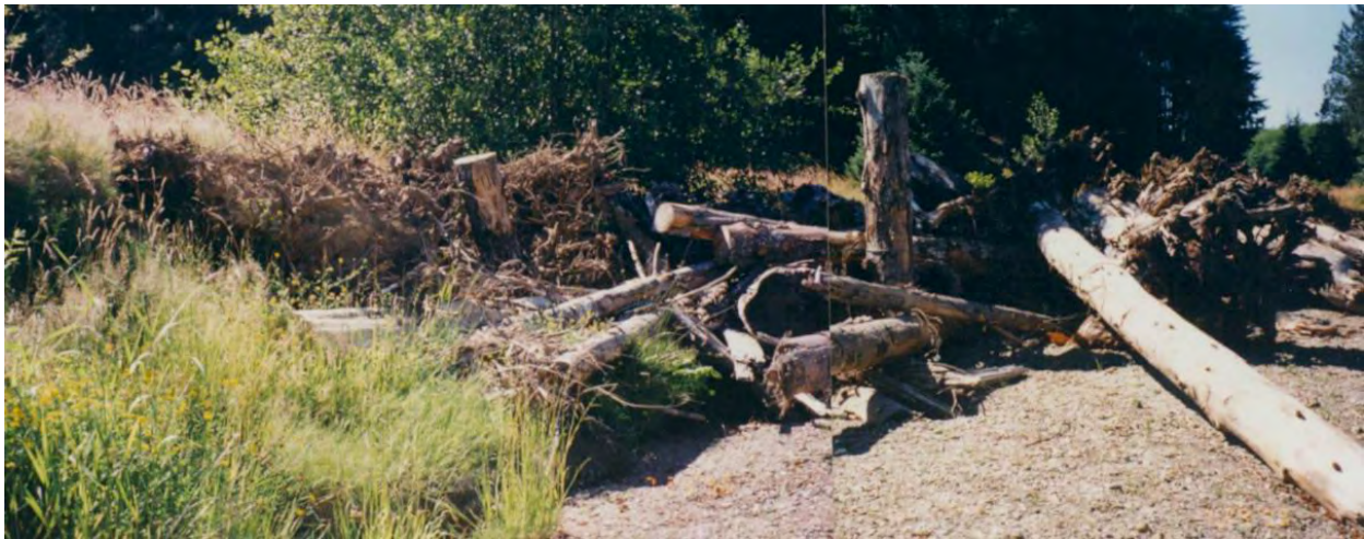
Large Wood and Log Jams Figure 19. A logjam anchored by driven log pilings on the Little Hoko River, Clallam County, Washington.
