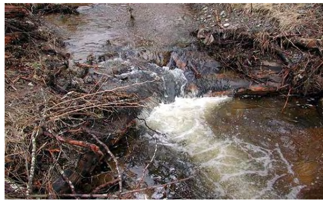
Large Wood and Log Jams Figure 17. A V-shaped log sill created with two crossed logs: (a) concept sketch showing small wood on upstream side of log to retain streambed sediment; (b) photo of crossed log structure (unidentified creek near Pysht River, Clallam County, Washington).
