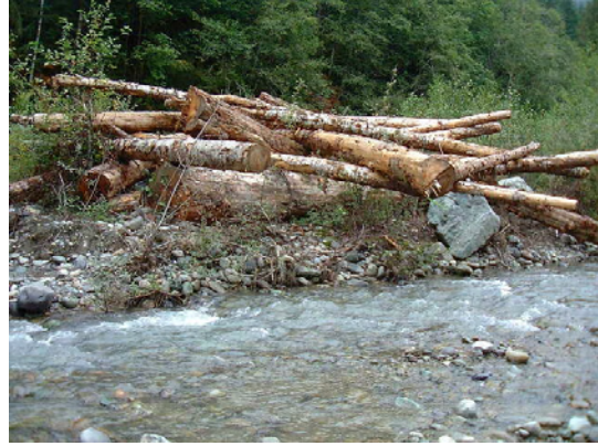
Large Wood and Log Jams Figure 3. LW placed on the floodplain will provide low velocity refuge during high flows. (Finney Creek, Skagit County, Washington).
