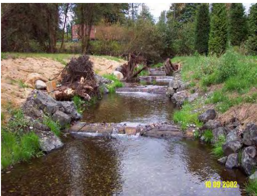
(e) Log weir grade controls. Hylebos Cr.
