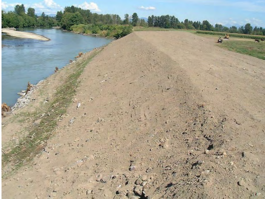
Figure 2.26. Dikes have been used throughout history to disconnect channels from their floodplains.
