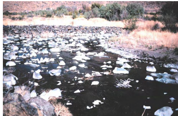
Boulder Clusters Figure 11: Constructed boulder clusters in Murderers Creek.
