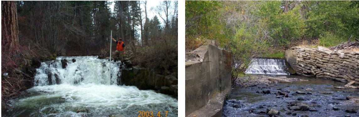
Figure 2.25. a) Natural fish passage barrier. b) Human-created fish passage barrier.
