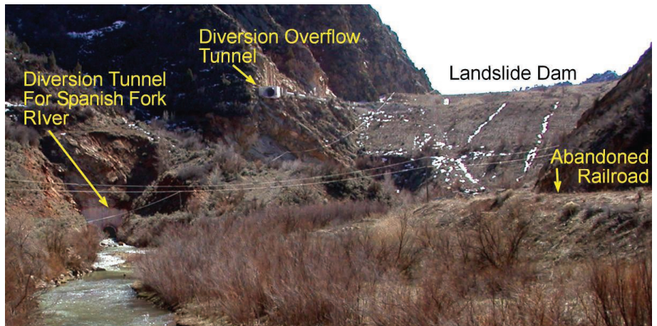
Figure C54. Closeup view of mitigation measures taken to reduce the impact of the Thistle landslide dam, showing the tunnel for the river, and the diversion overflow tunnel. (Photograph courtesy of the Utah Geological Survey).
