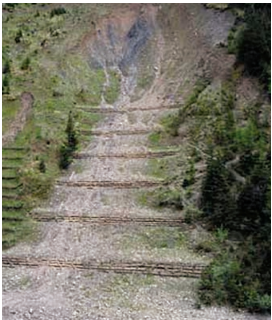
Figure C7. Schematic and photograph of a crib wall check dam, which is one kind of check dam. (Graphic from Reference 11, photograph taken in Trafoi, Italy, courtesy of "Erosion Control," Forester Communications, Santa Barbara, California, USA.)
