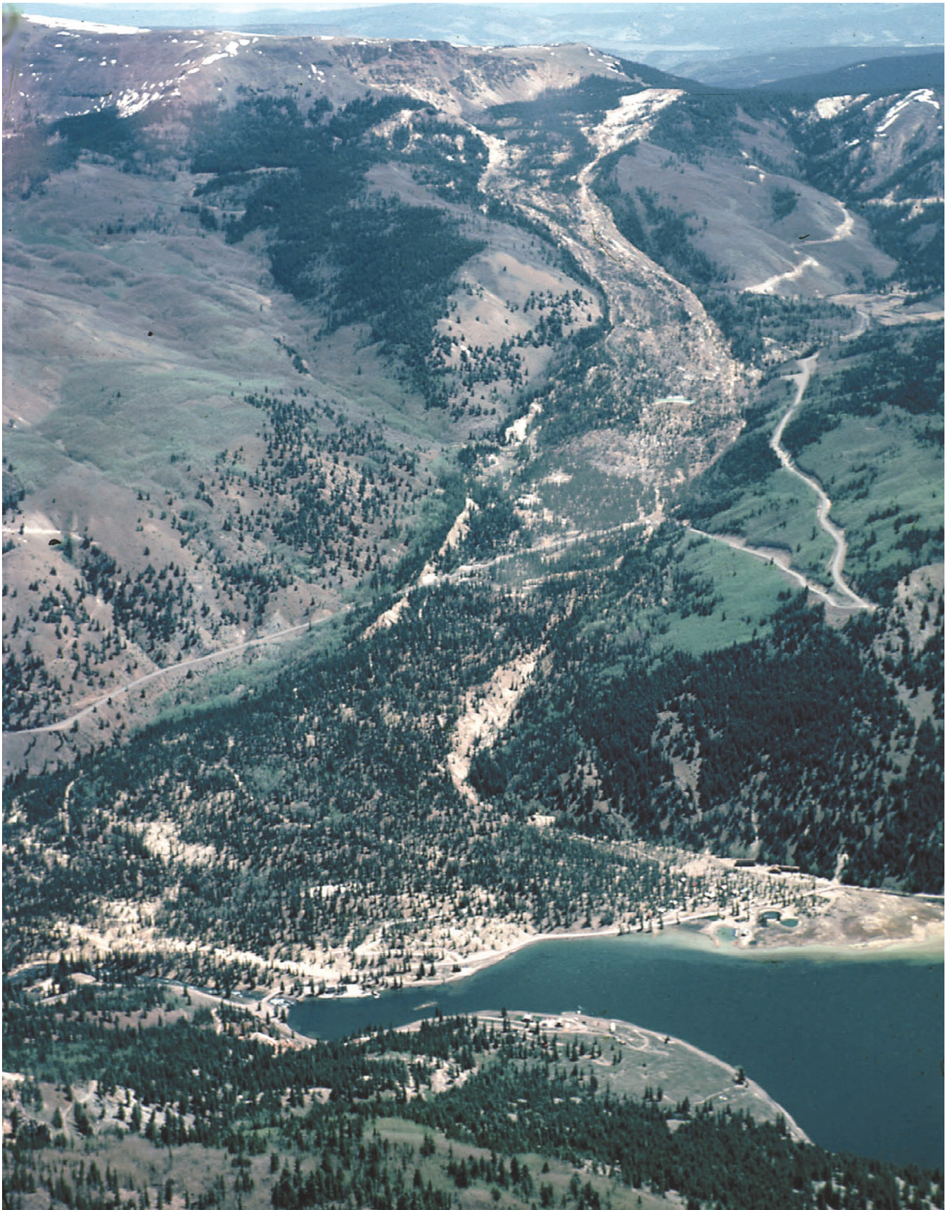
Figure 32. The Slumgullion landslide, Colorado, USA. This landslide (formally referred to also as an earthflow) dammed the Lake Fork of the Gunnison River, which flooded the valley and formed Lake Cristobal. (Photograph by Jeff Coe, U.S. Geological Survey.)
