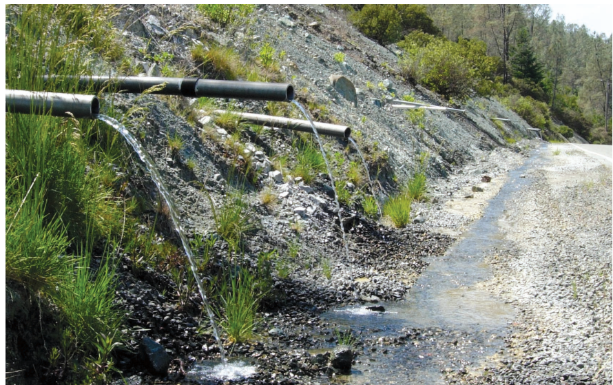
Figure C10. Schematic of drainpipes. (Schematic from Reference 11.) Photograph of drainpipes in a landslide in California, USA, by Andrew Alden.
