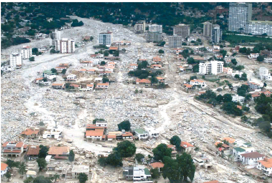
Figure 14. Debris-flow damage to the city of Caraballeda, located at the base of the Cordillera de la Costan, on the north coast of Venezuela. In December 1999, this area was hit by Venezuela's worst natural disaster of the 20th century; several days of torrential rain triggered flows of mud, boulders, water, and trees that killed as many as 30,000 people. (Photograph by L.M. Smith, Waterways Experiment Station, U.S. Army Corps of Engineers.)
