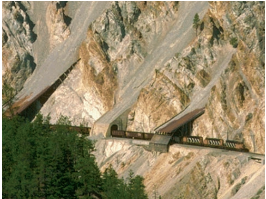
Figure C24. Pitquah rock sheds, British Columbia, Canada. These sheds enclose sections of railroad, protecting it from rockfall and rock avalanches. (Photograph by John Carter, www.trainet.org .)
