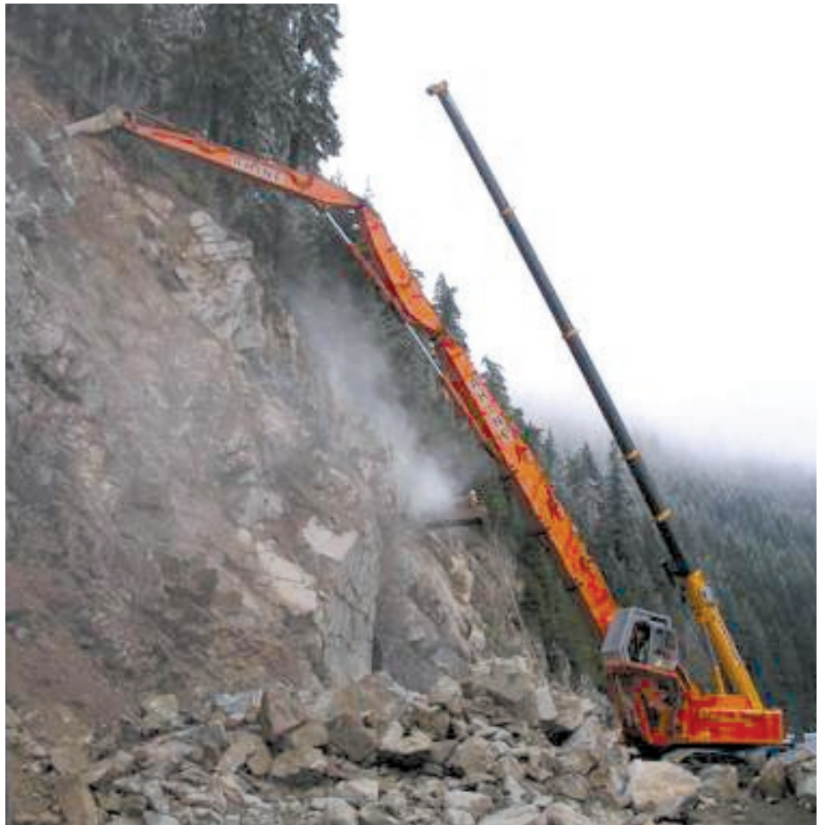
Figure C30. A hydraulic rock hammer in action, bringing down rock from the slope. This is an alternative to blasting rocks down. (Photograph by Washington Department of Transportation, USA.)
