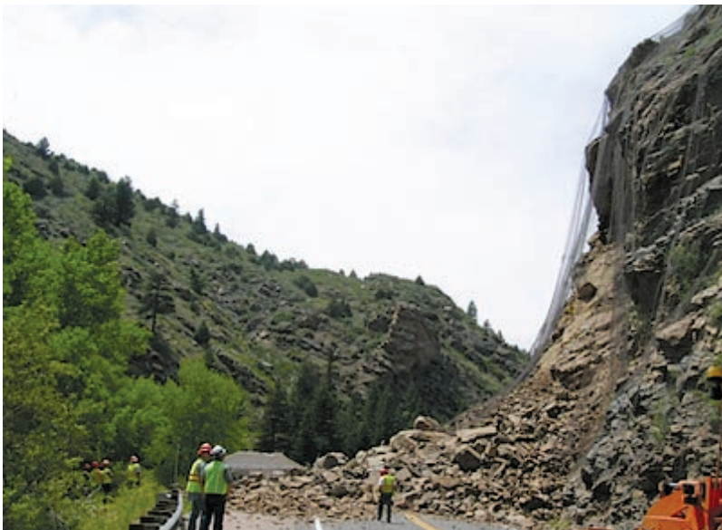
Figure 4. A rockfall/slide that occurred in Clear Creek Canyon, Colorado, USA, in 2005, closing the canyon to traffic for a number of weeks. The photograph also shows an example of a rock curtain, a barrier commonly applied over hazardous rock faces (right center of photograph). (Photograph by Colorado Geological Survey.)
