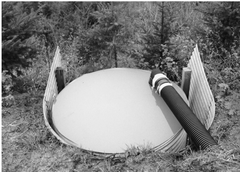
Figure 3. Photograph of sediment trap with crossdrain outlet.
