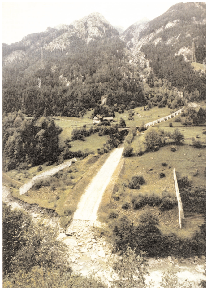
Figure 31. Clear-span bridge constructed in Canton of Bern, Switzerland, along with guidewalls and a concrete-lined channel. (Photo from United Nations, 1996)
