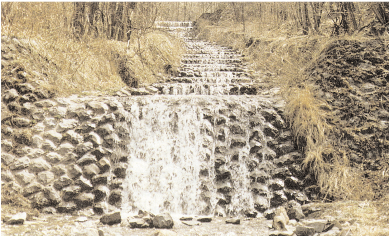
Figure 30. Ground sills constructed in Nagano, Japan. (Photo from United Nations, 1996)
