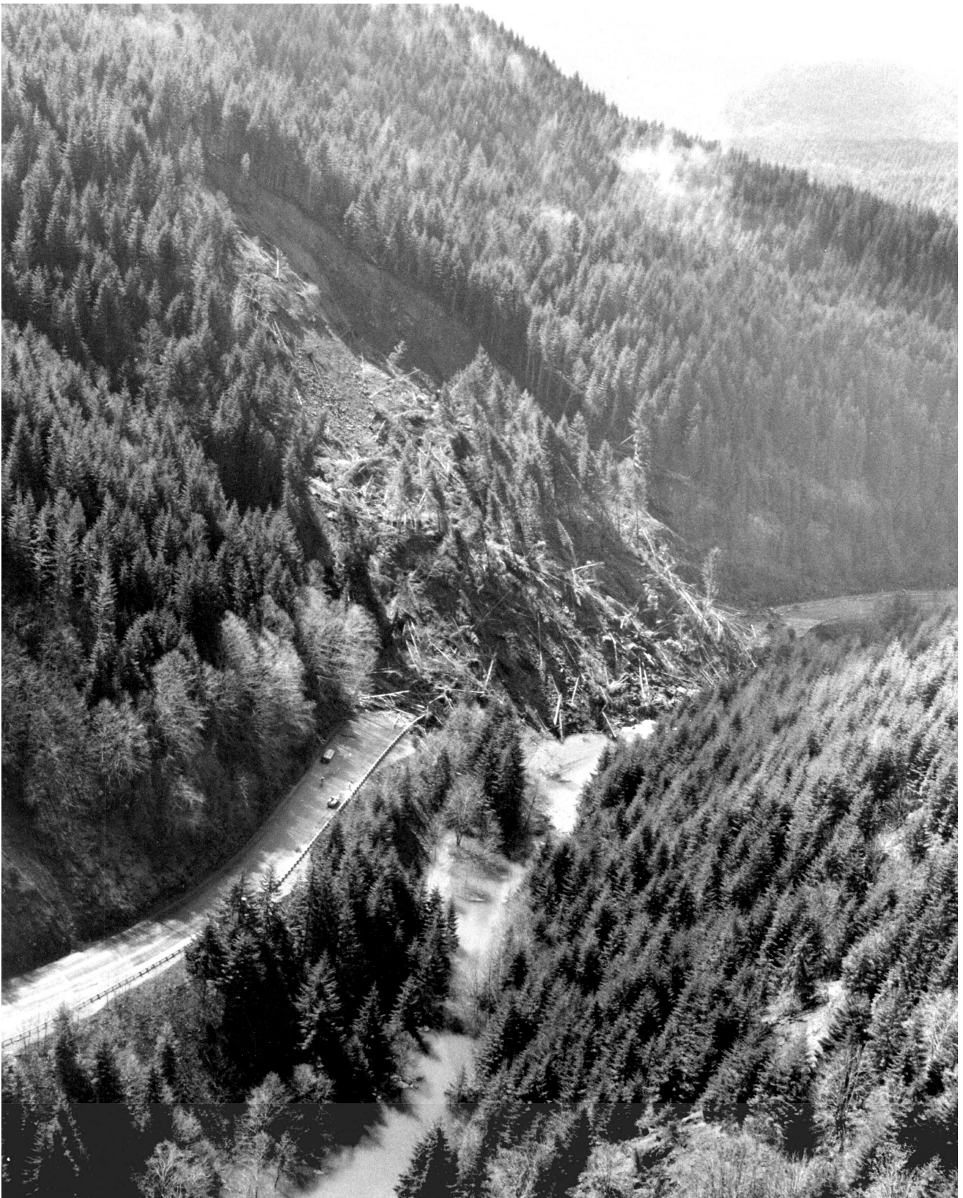
Figure 4. Rockslide that occurred along the Wilson River Highway (Hwy 6) in 1991. Though not a debris flow, this hazardous area is identified by the hazard model. (Photo courtesy of Susanne L. D’Agnese, Oregon Department of Transportation)
