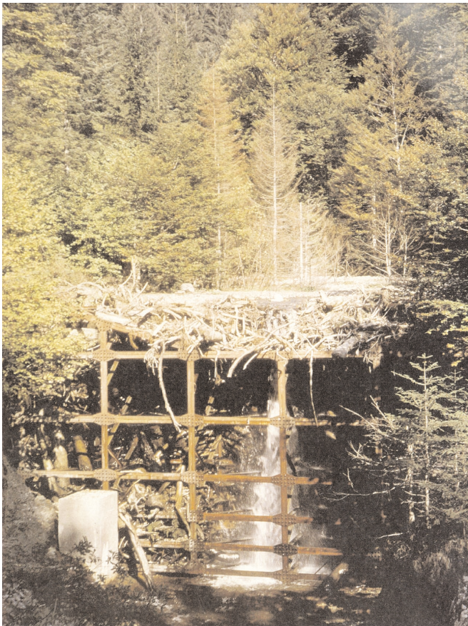
Figure 29. Steel-lattice dam constructed in Kirchbachgraben, Austria. (Photo from United Nations, 1996)
