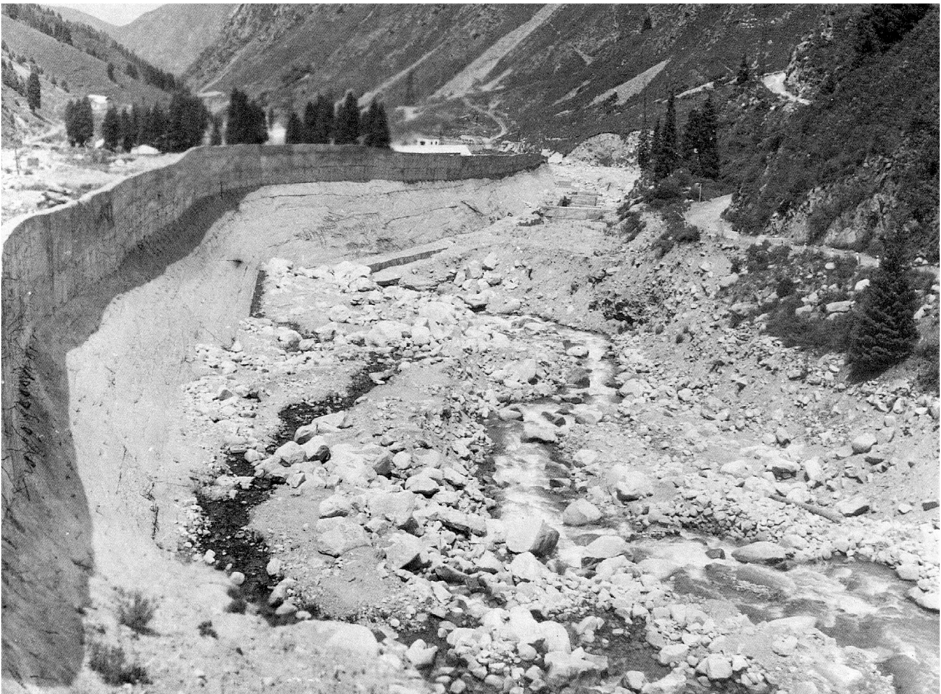
↑ Figure 34. Protection wall constructed on the Bolshaya Almatinka River, Kazakhstan. (Photo from United Nations, 1996)
