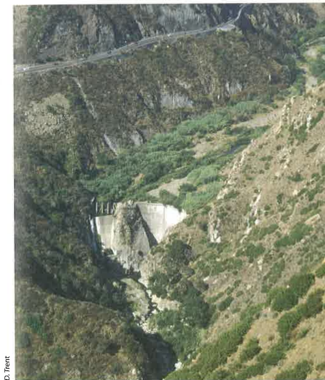
PHOTOGRAPH 7.25 Sediment Stored Behind Dam. The 30-meter-tall Rindge Dam is located in Malibu, California. The main arch of the dam was completed in 1924 but now the reservoir is completely filled with sediment from the steep, rapidly eroding watershed. Fish advocates have called for the dam's removal because it is blocking steelhead trout from accessing the upper reaches of Malibu Creek.
