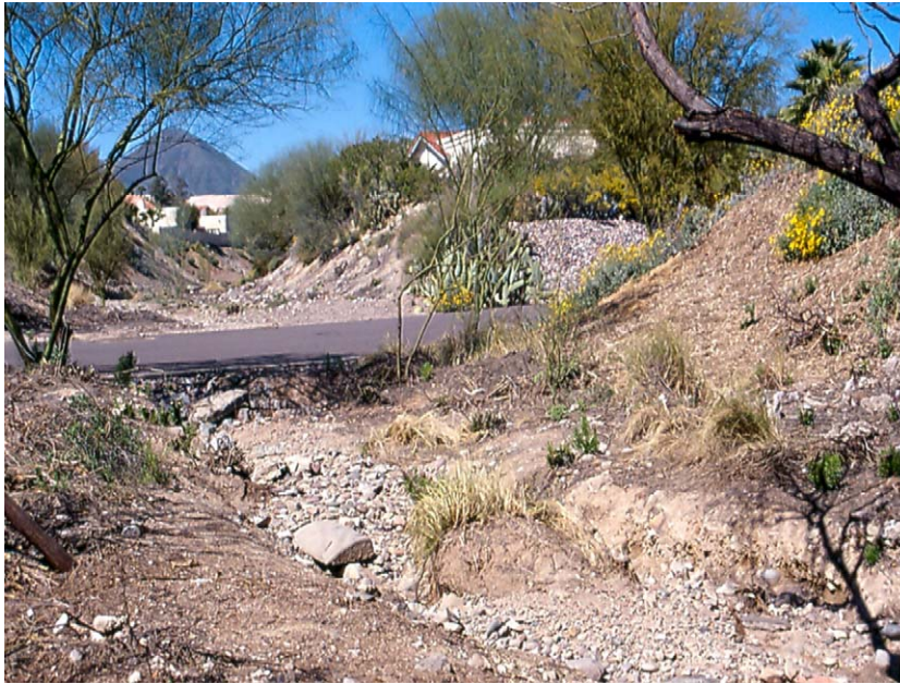
Fig. 9. Representative channel in Fountain Hills, Arizona, crossed by repeating system of roads. The spatially varied response is characterized by incised river channels downstream of road crossings with low width–depth ratios, and aggraded wide and shallow cross sections upstream (see Chin and Gregory, 2001; photograph by A. Chin).
