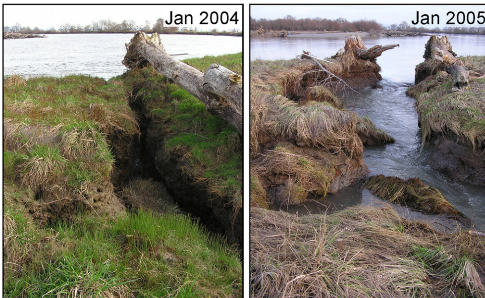
Fig. 2. Left photo: upstream end of an 11-m-long newly incised avulsion channel (foreground) connecting the North Fork Skagit River (background) to a previously blind tidal channel (not in the frame). Right photo: the same channel one year later. The log on the right bank is the same in both photos and indicates relative scale. The upstream end of the channel is 0.7 m wide in 2004 and 2.5 m wide in 2005. In January 2010, the most recent observation, it was 13 m wide.
