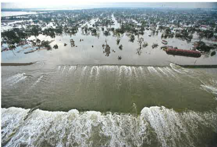
(d) Water flowing across the levees bordering the 17th Street Canal after the hurricane had passed.
