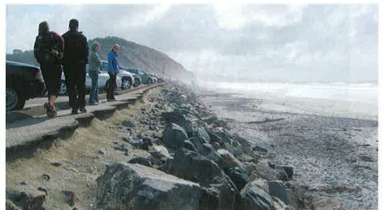
(d) Riprap will slow erosion of a parking lot along a California beach.
