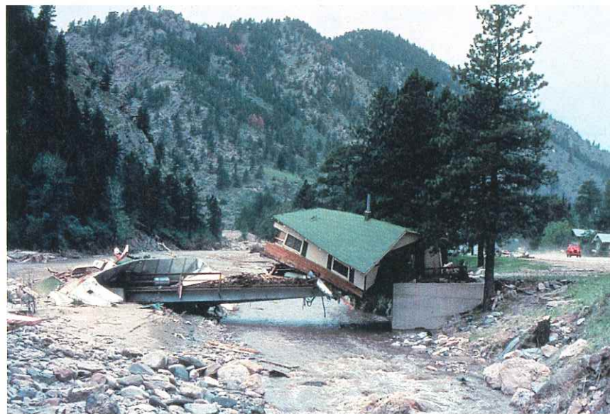
(b) During the 1976 Big Thompson River flash flood, this house was carried off its foundation and dropped on a bridge.
