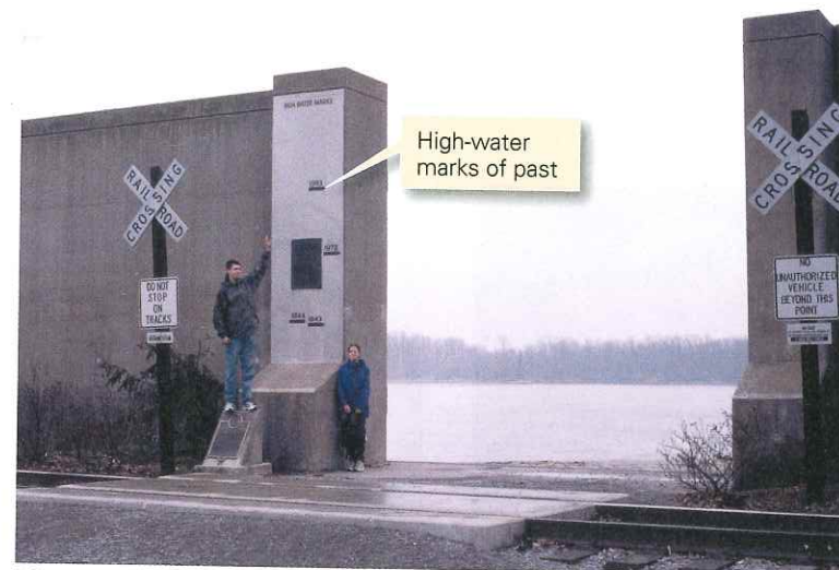
(c) A concrete floodwall at Cape Girardeau, Missouri. When floods threaten, a crane drops a gate into the slot to hold out the river.
