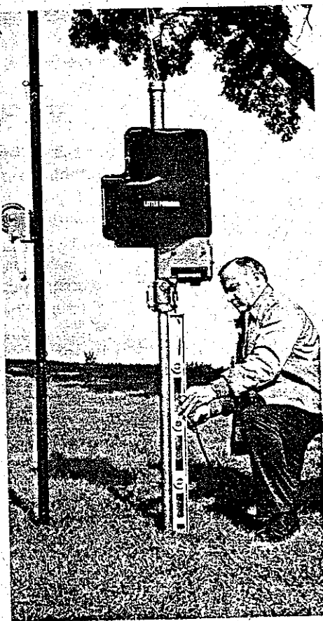
Figure 10.53. A mechanical driving device facilitates placing a large number of well points. (Crystal Water Products)
