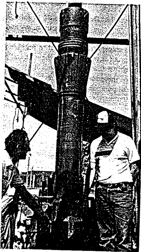
Figure 10.58. A cement basket is mounted on the casing to support the column of cement grout to be placed above it. Use of a basket prevents grout from entering weak underlying formations or infiltrating the filter pack. (Corner S. A.)
