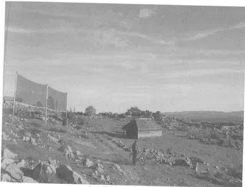
FIG. 2.13 Fog collection system on a farm in Tojquia, Guatemala. The vertical mesh panels capture atmospheric moisture and allow it to trickle into the tank at the base of the collectors. The system provides drinking water and other uses for the community.
