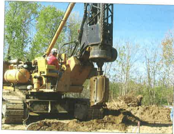
Figure 7.22. Bucket auger drilling rig (Powers et al. 2007).
