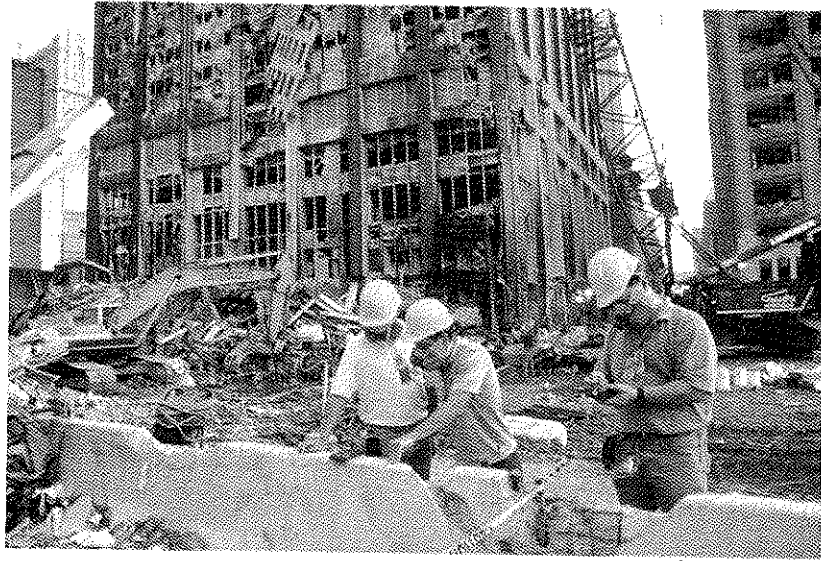
FIGURE 9.19: Hand-held GPS data collection suffered from multipath signal deflections from the considerable amount of metal.
