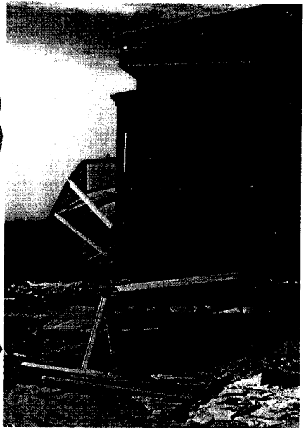
Figure 31. Construction (above) and destruction (below) of condominium built in 1982 and small remnant of marine terrace at Jump-Off Joe. From Sayre and Komar (1988).
