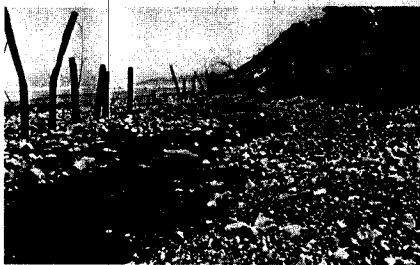
Figure 28. Progressive erosion of Cape Lookout State Park following the 1982-83 El Niño. (upper) Destruction of log bulkhead and initiation of dune erosion during October 1984. (lower) Erosion during winter of 1988, leaving a beach composed of cobbles and gravel rather than sand, and I-beams of log bulkhead at mid-beach. From Komar and others (1988).
