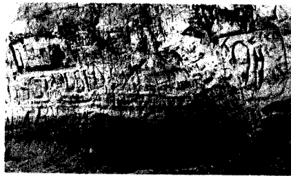
Figure 30. Retreat of bluff in Lincoln City caused by children carving graffiti and digging caves.
