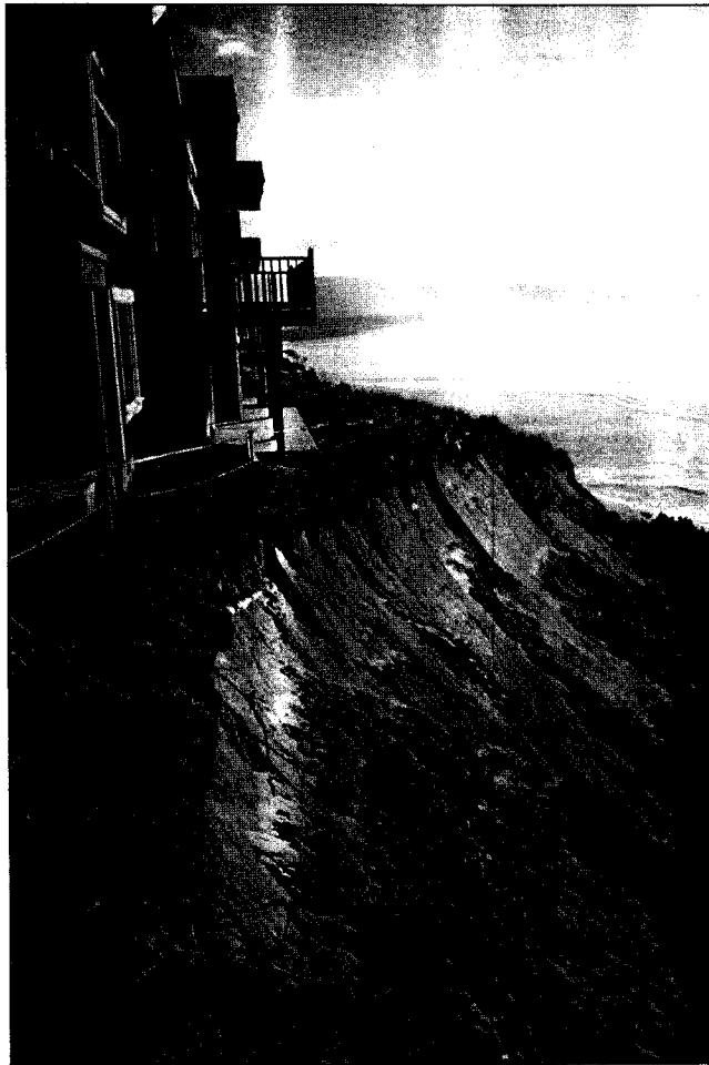
Figure 10. Homes at The Capes. Erosion of the toe of the landslide during the 1997-98 El Niño winter has caused the slide to become unstable, and slippage is threatening the first line of homes.
