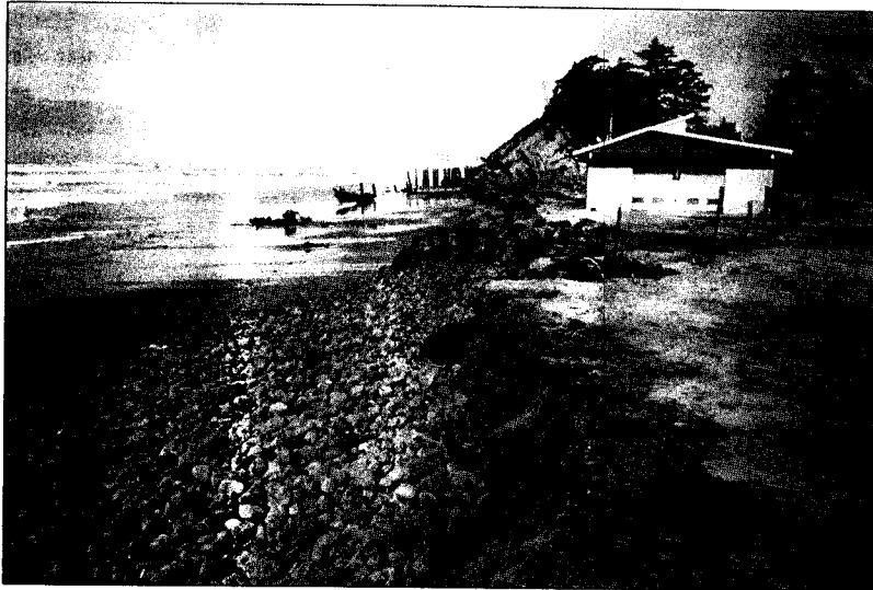
Figure 8. Recent erosion at Cape Lookout State Park on Netarts Spit has cut back the large coastal dunes and is now eroding the campground.
