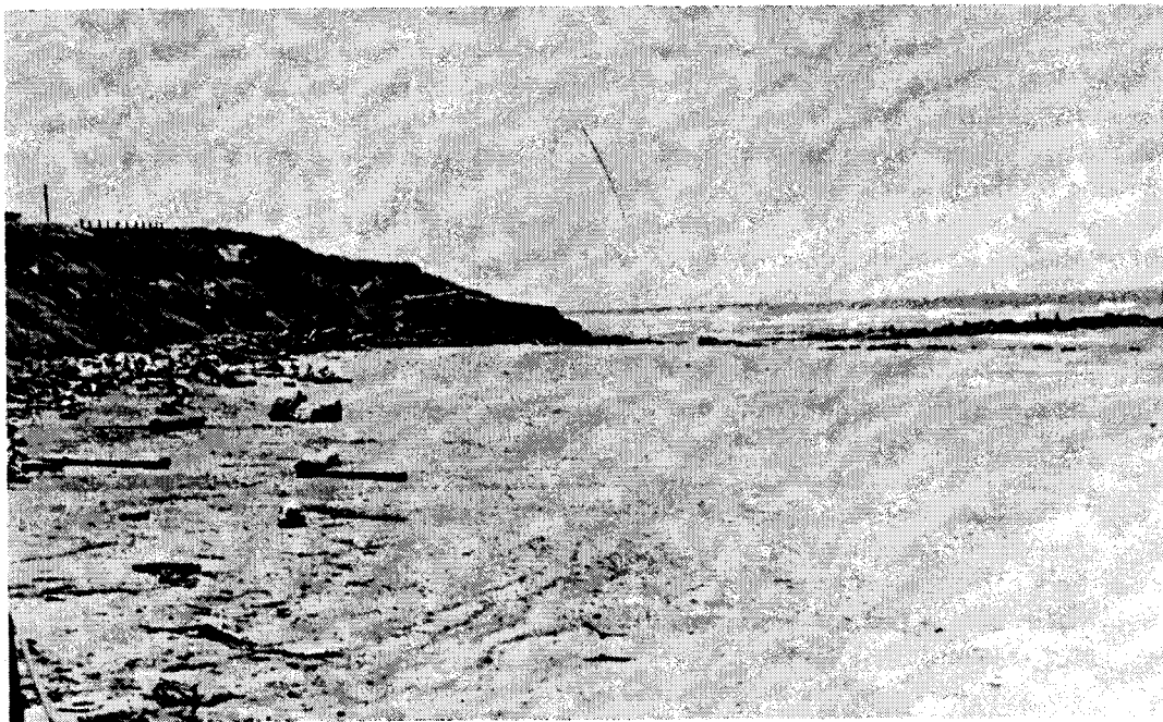
Photo 62. Photo taken from approximately same location in 1973 shows amount of recession of small headland and its terrace platform.
