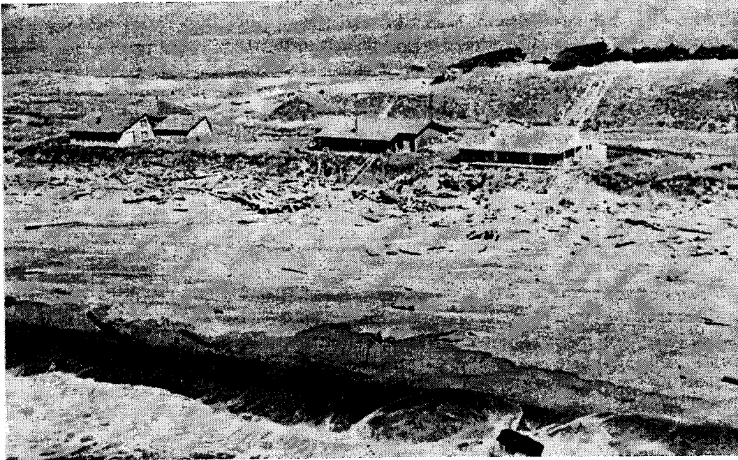
Photo 63. Some of the houses built on the low dunes of Siletz spit. Photo taken in fall of 1972 before severe erosion of spit by winter storms.
